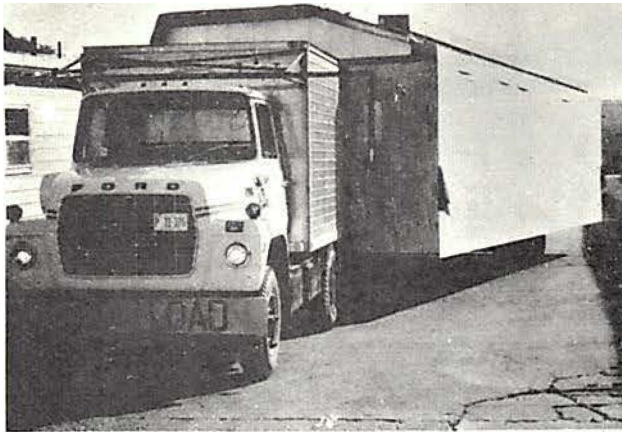
Figure 4. Typical 14-foot wide modular section.
