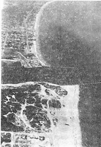
FIGURE 2 - View, looking West, of Jetties at Little Creek. The net sand drift is to the West. Note the offset in beach width caused by the trapping action of the long east Jetty with resulting starvation of the beaches to the west.
