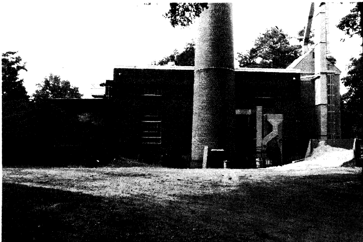
Figure C-4. The heating plant at Piedmont Geriatric Hospital. Coal storage can be seen at the left hand side of the photo. The wood-waste fuel delivery hopper and the fuel storage silo can be seen on the right.
