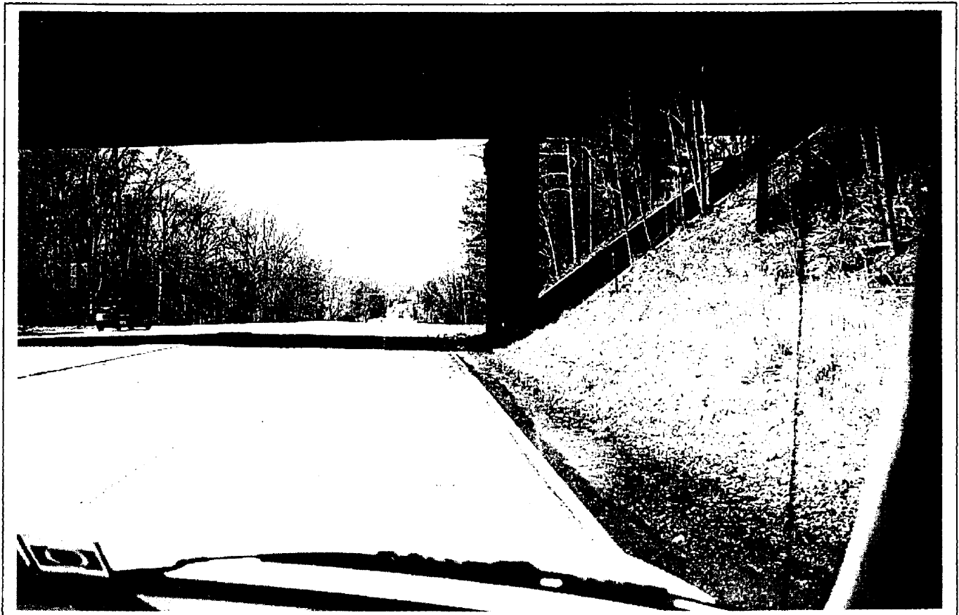
Fixed objects near the roadway, such as the bridge pier shown here, present potential safety hazards.
