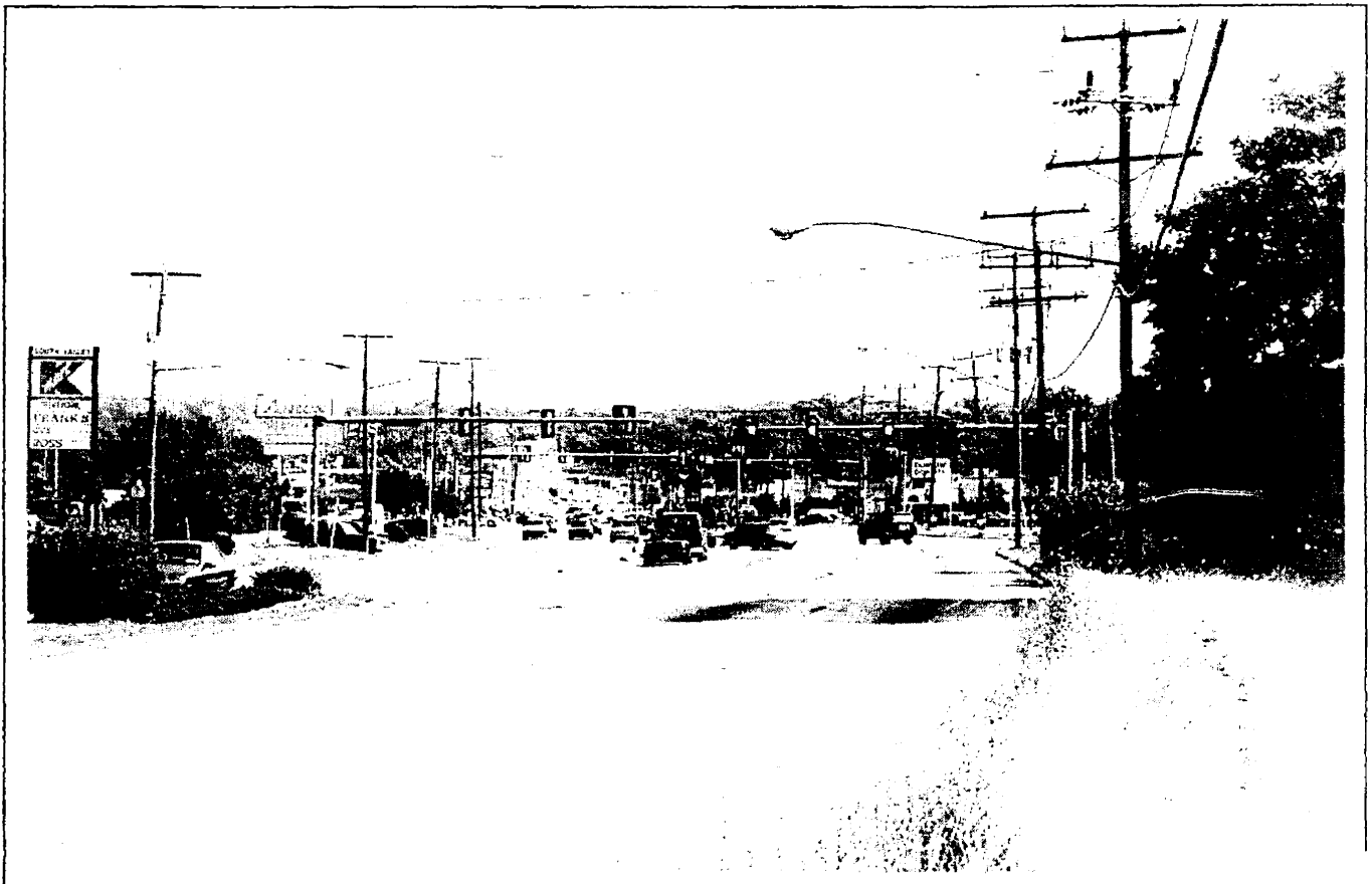
View looking north on Route 1 toward Fordson Road in Hybla Valley
