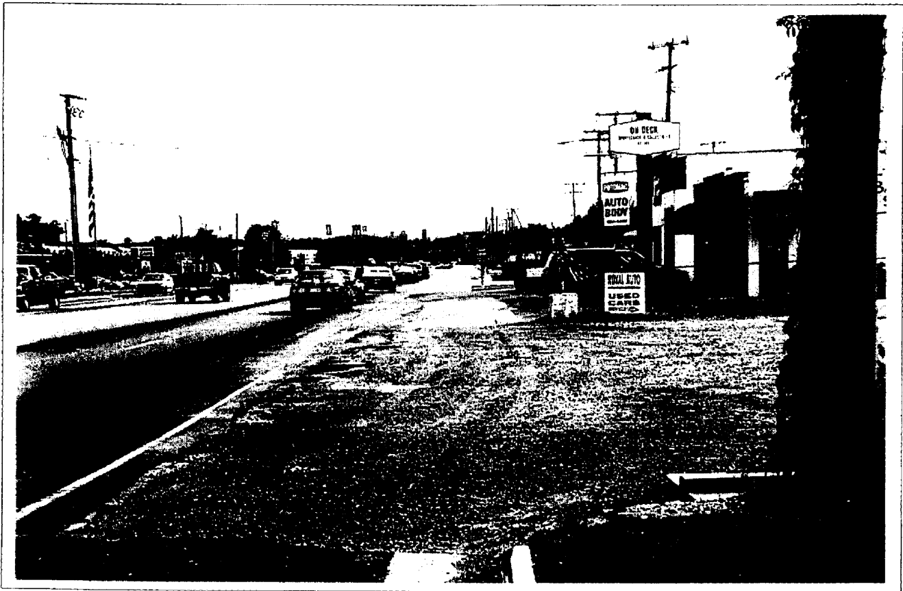
Lack of access control and lack of a consistent road edge treatment contribute to a negative image due to poor appearance and numerous traffic conflict points.
