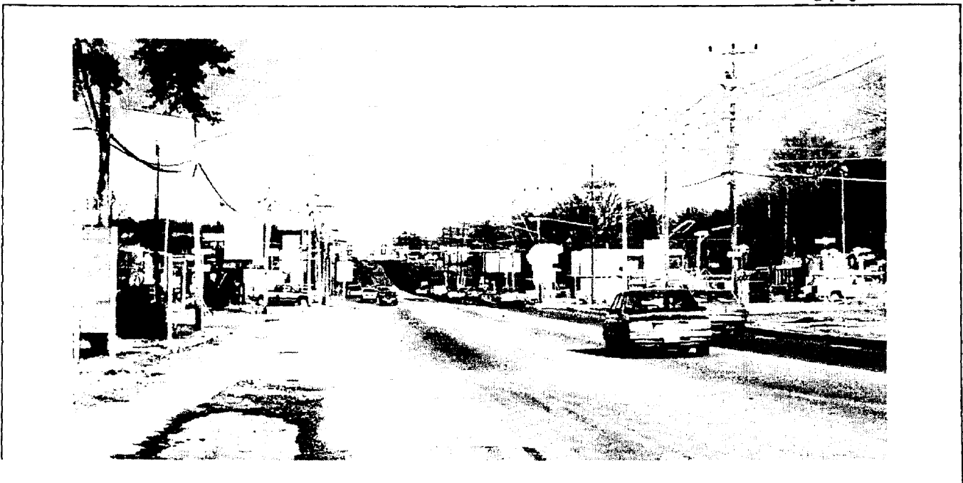
Most of Route 1 has received only spot intersection and frontage improvements over the last 30 to 40 years.
