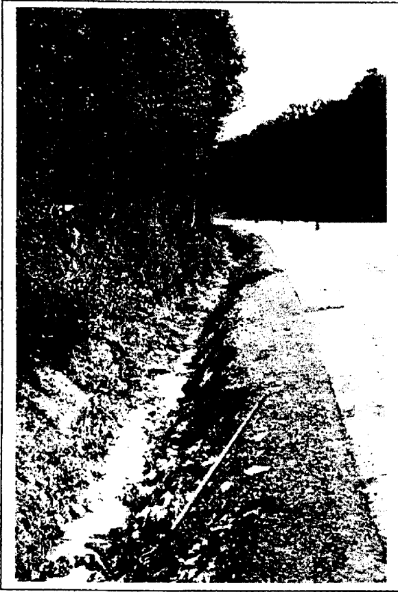
Many ditches are eroding to the point of destabilizing shoulders and guardrail posts.
