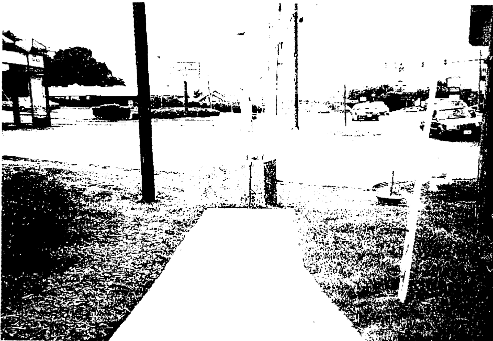
Many of the sidewalks along Route 1 are discontinuous or have obstructions blocking them. Here the sidewalk ends at an obstruction.
