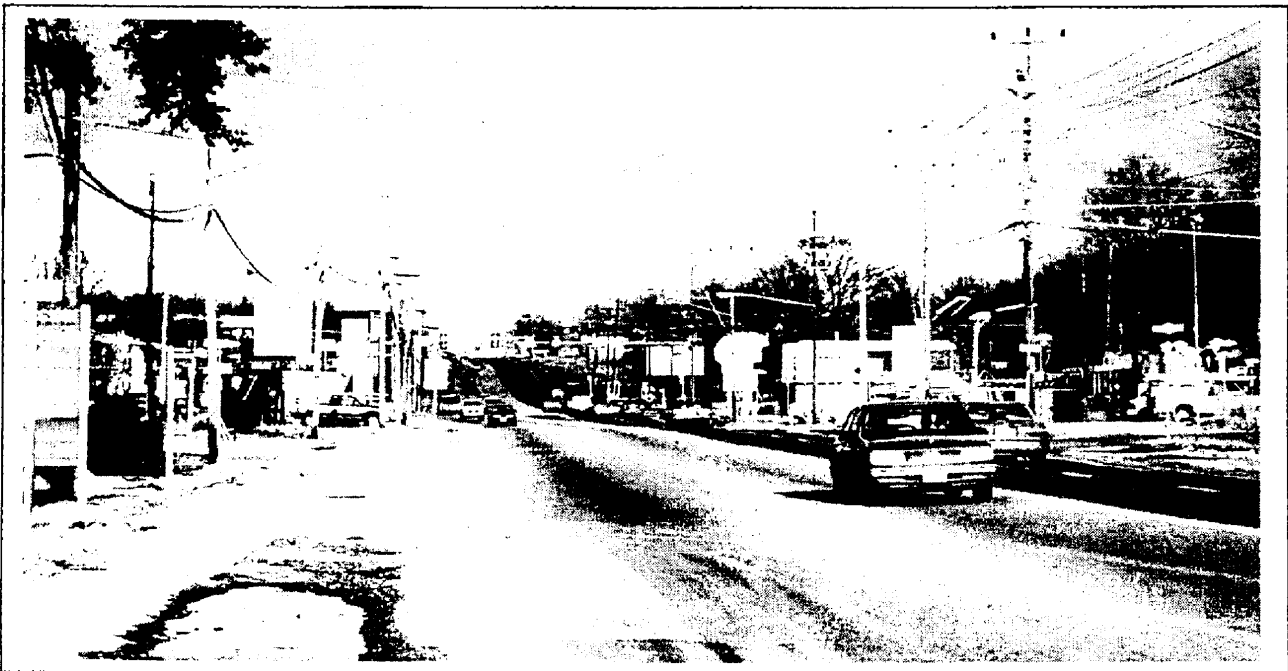
Much of Route 1 has inconsistent cross-sections and lacks left turn lanes.
