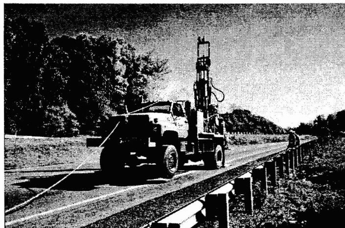
Photo 7. VDOT Drill Rig
