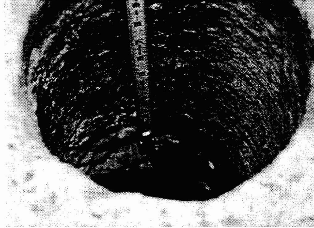
Photo 10. Base Course Thickness Measurement Through Core Hole
