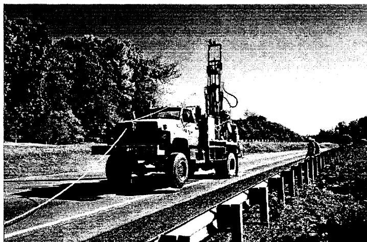
Photo 7. VDOT Drill Rig
