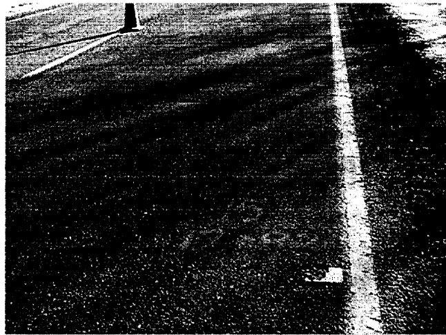
Photo 3. Photographic Documentation of Site 15. Note the segment's unique identification number and the transverse crack.
