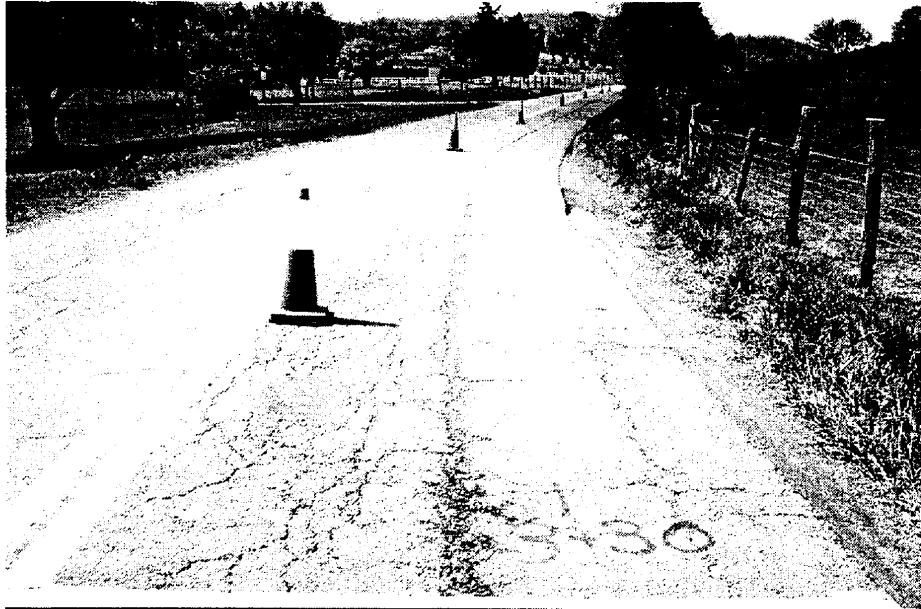
Photo 15. Severe Fatigue Damage with Patched Pothole at Site 1: Route 607, Wythe County, April 2000
