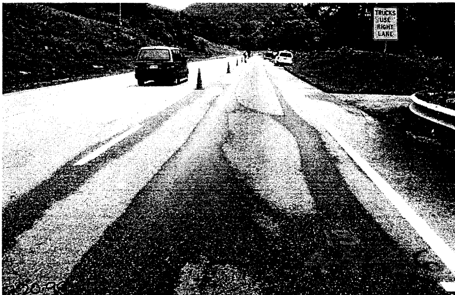
Photo 18. Wheel Path Rutting at Site 13: Route 58, Lee County, July 1999. Note standing water in wheel paths.
