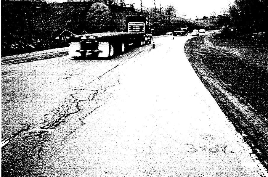
Photo 17. Moderate Fatigue Damage at Site 18: Route Alternate 58, Russell County, April 2000
