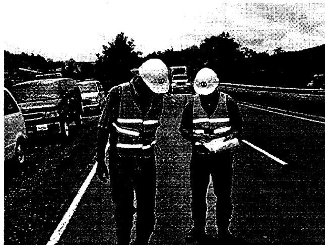
Photo 2. Distress Identification and Documentation During Visual Survey
