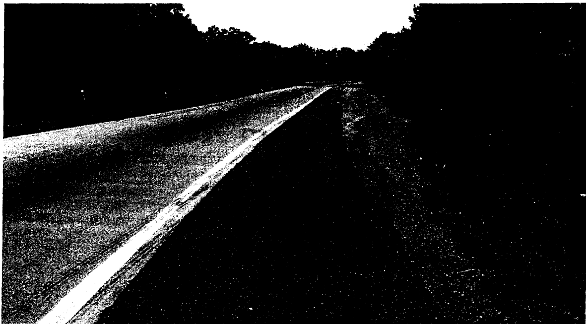
Figure 4. Case Study 1: View Looking West, the Direction in Which Involved Trucks Were Traveling, at Ramp. Photo was taken about 500 feet before the point of collision.
