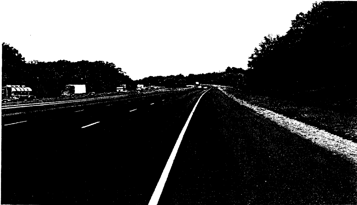
Figure 11. Case Study 3: View Looking North in Direction in Which Fire Trucks Were Traveling. Note the rumble stripping.
