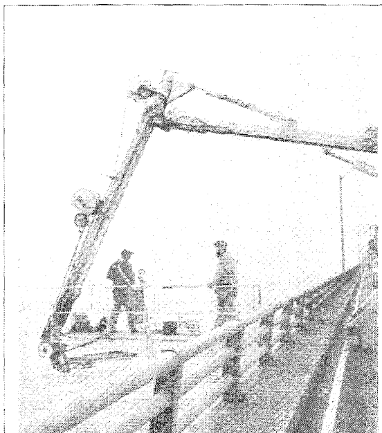
Repairing concrete from the Snooper.
