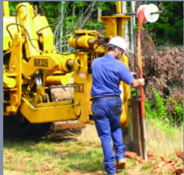
Cable plow installing fiber optic cable.
