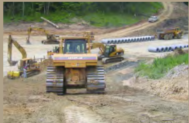
Site preparation at Duffield Regional Industrial Park.
