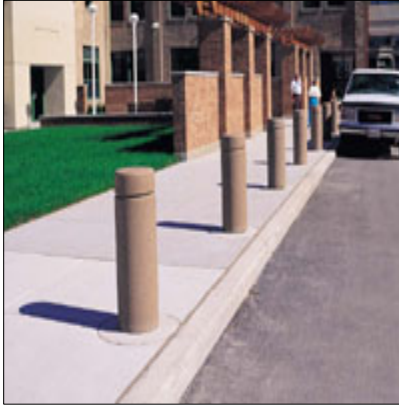
Bollards deter vehicle access
