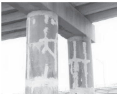
These pilings, damaged in construction, have been repaired.
