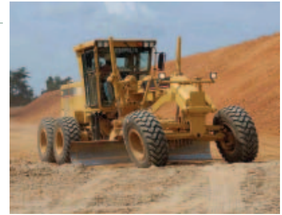
SsVCC heavy duty equipment operator training program
