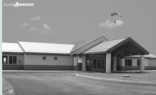
The Middle Peninsula Airport Authority borrowed through the Airports RLF to fund the construction of an aviation terminal building.
