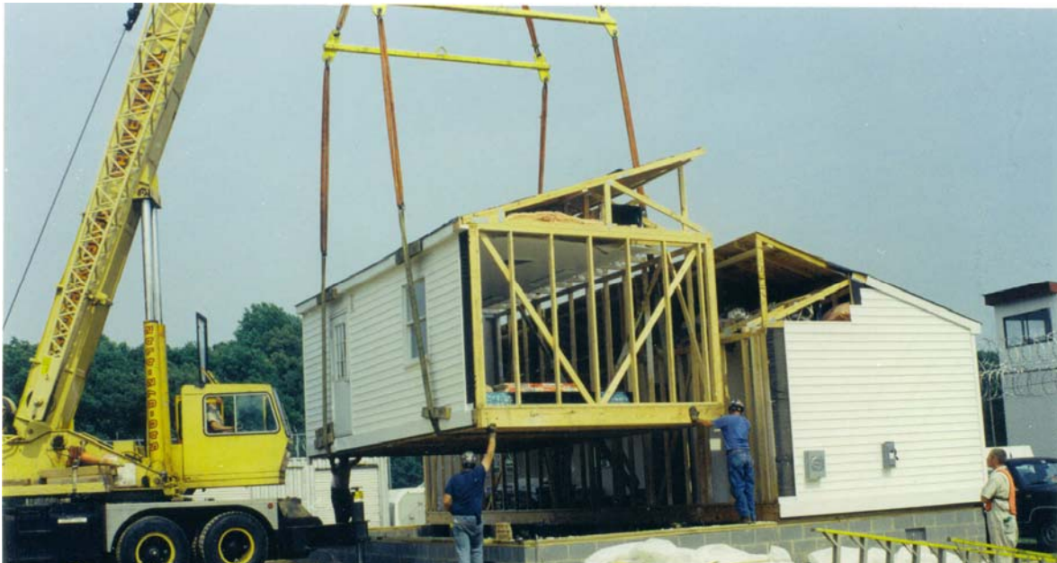
Modular Classroom Being Placed on Foundation
