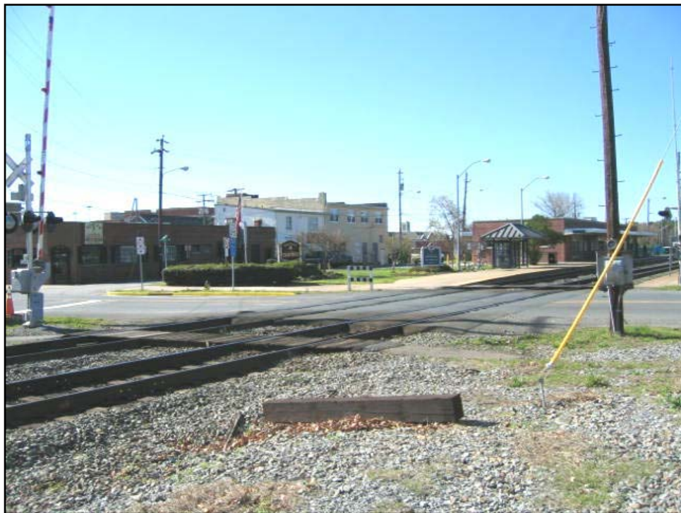
Photo 4-7: Existing two-track public roadway grade crossing (Potomac Avenue in Quantico) which will require signal relocation.
