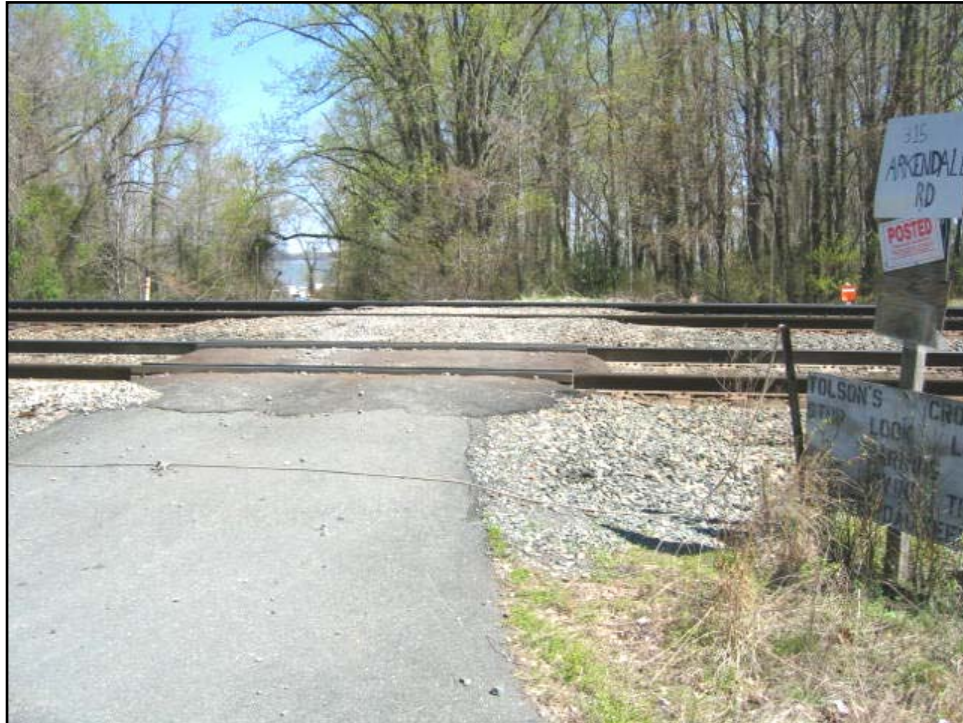
Photo 4-8: Private roadway grade crossing over CSX tracks. Note there are no gates or flashing lights.
