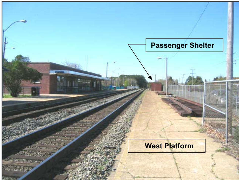
Photo 4-11: Station and platforms at Quantico Station. Third track construction will require demolition and reconstruction of the west platform and demolition of the passenger shelter.
