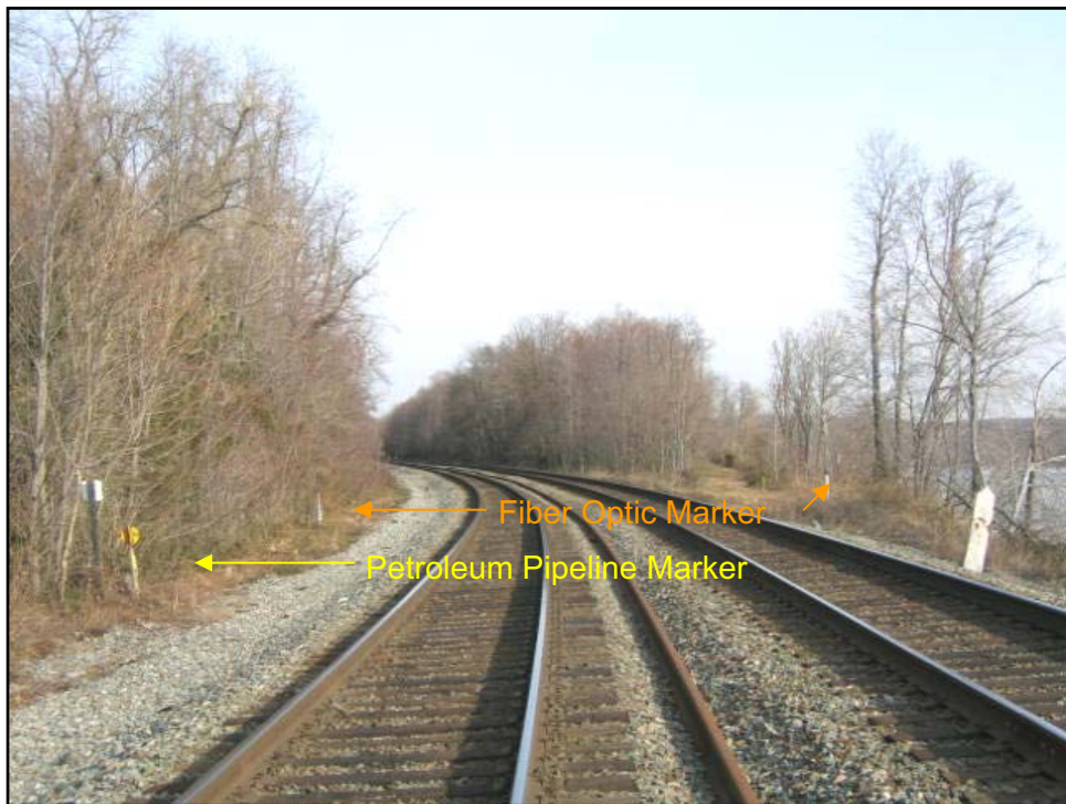
Photo 4-9: View of track looking north near MP 83. Note both petroleum pipeline and fiber optic cable markers.
