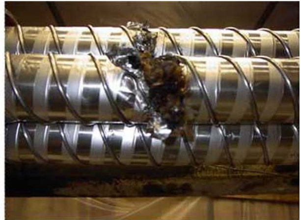
Damaged Insulation on Same Cable
