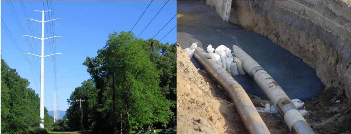
Figure 1: Overhead and Underground Electric Transmission Lines in Virginia
