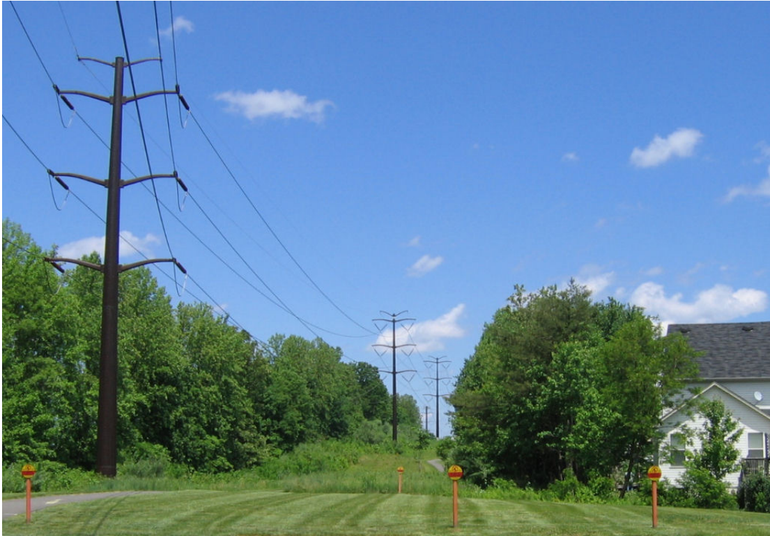
Figure 2: Overhead 230 kV Transmission Towers, With Two Transmission Lines, Along a Natural Gas Pipeline in Fairfax County
