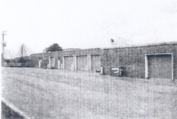
Detached Service Building, 13,500 s.f on two floors
