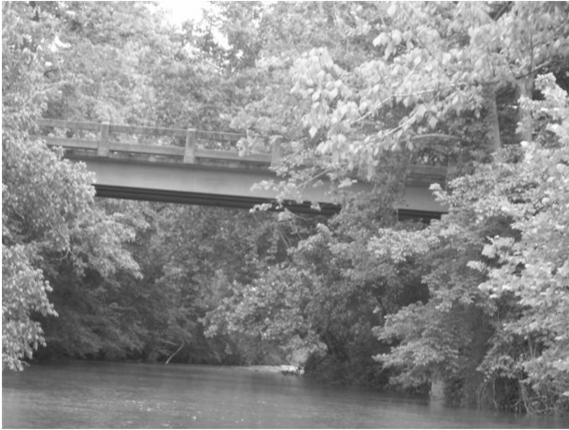
Figure 7 Route 695 bridge crossing the South Mayo River
