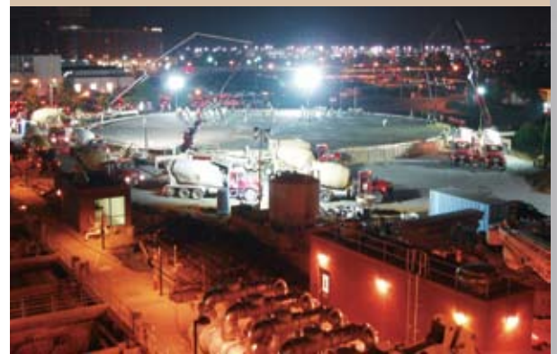
Arlington County wastewater treatment plant under construction.
