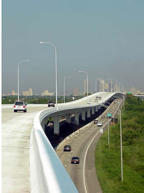
Figure 9 – Tampa Elevated Cashless ORT lanes
