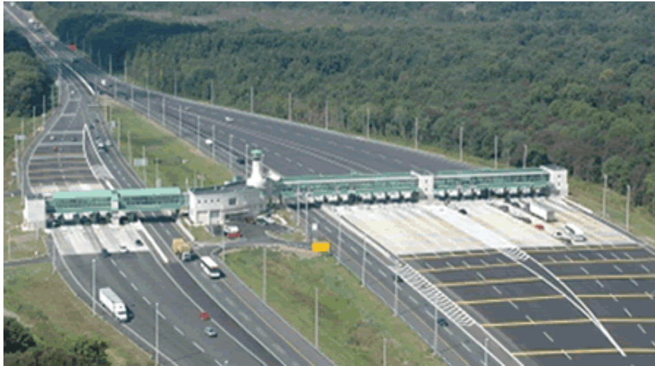
Figure 7 - New Jersey Mixed ORT/Cash toll plaza
