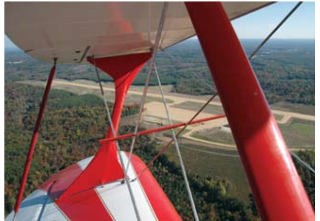
Tappahannock-Essex Airport under construction Credit: David Broad ©2007 Digital Wisdom Inc.
