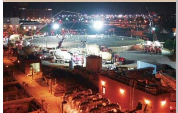
Arlington County wastewater treatment plant under construction.
