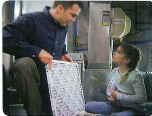
Video: man replacing a/c filter V/O: After replacing the filter
