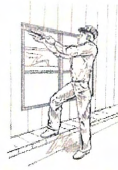
Download image in JPG formats Caulking around an exterior window
