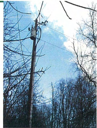
Trees within 10 feet of power lines can only be trimmed or removed by NOVEC contractors
