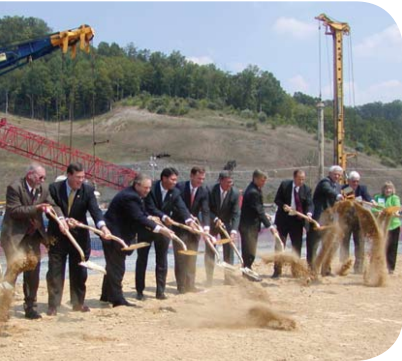
More than 300 persons attend the August 14 groundbreaking ceremony for Dominion Power's $1.8 billion Virginia City Hybrid Energy Center in Wise County, described as the largest economic development project in the history of the region.
