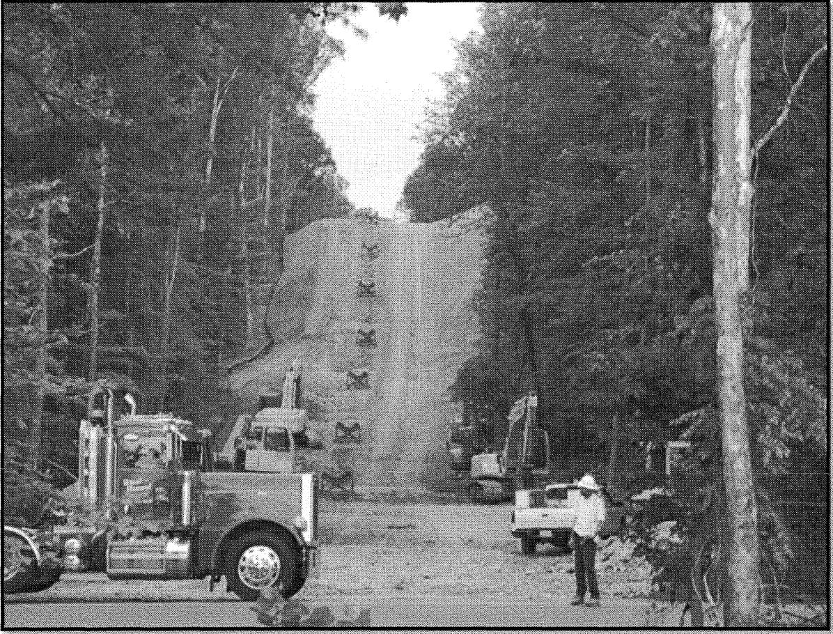
Figure 10: Cleared right of way for Garrisonville project.
