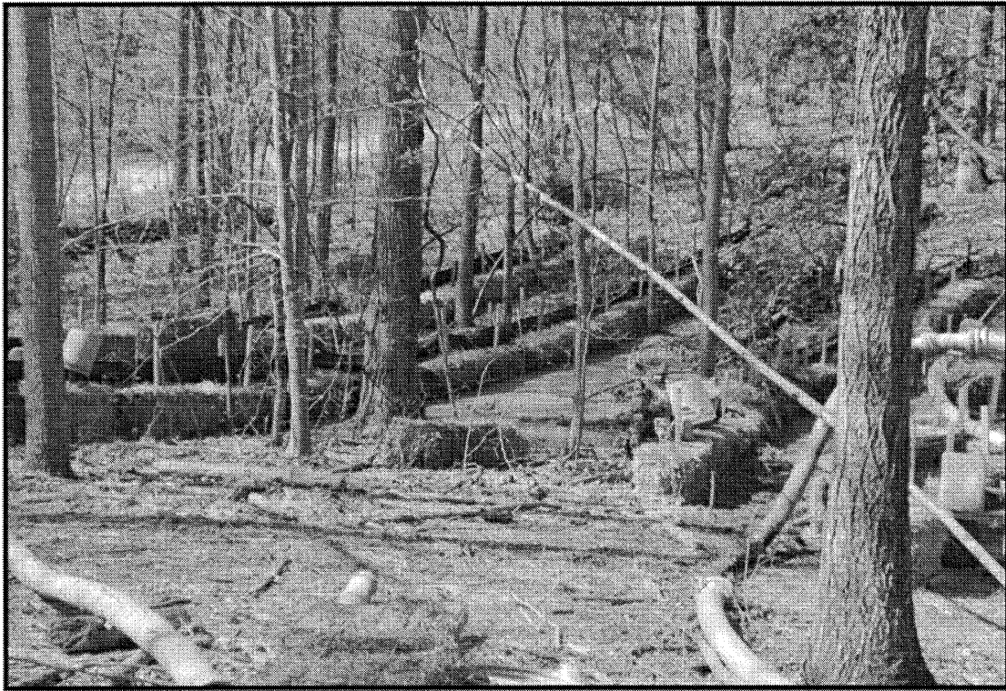
Figure 5: Site of frac-out showing containment measures for the protection of the environment.
