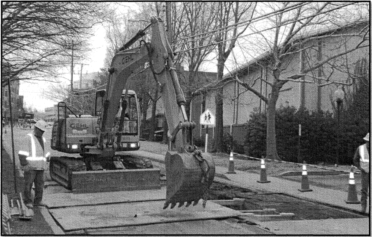
Figure 8: Excavation for Clarendon -- Ballston underground transmission line.
