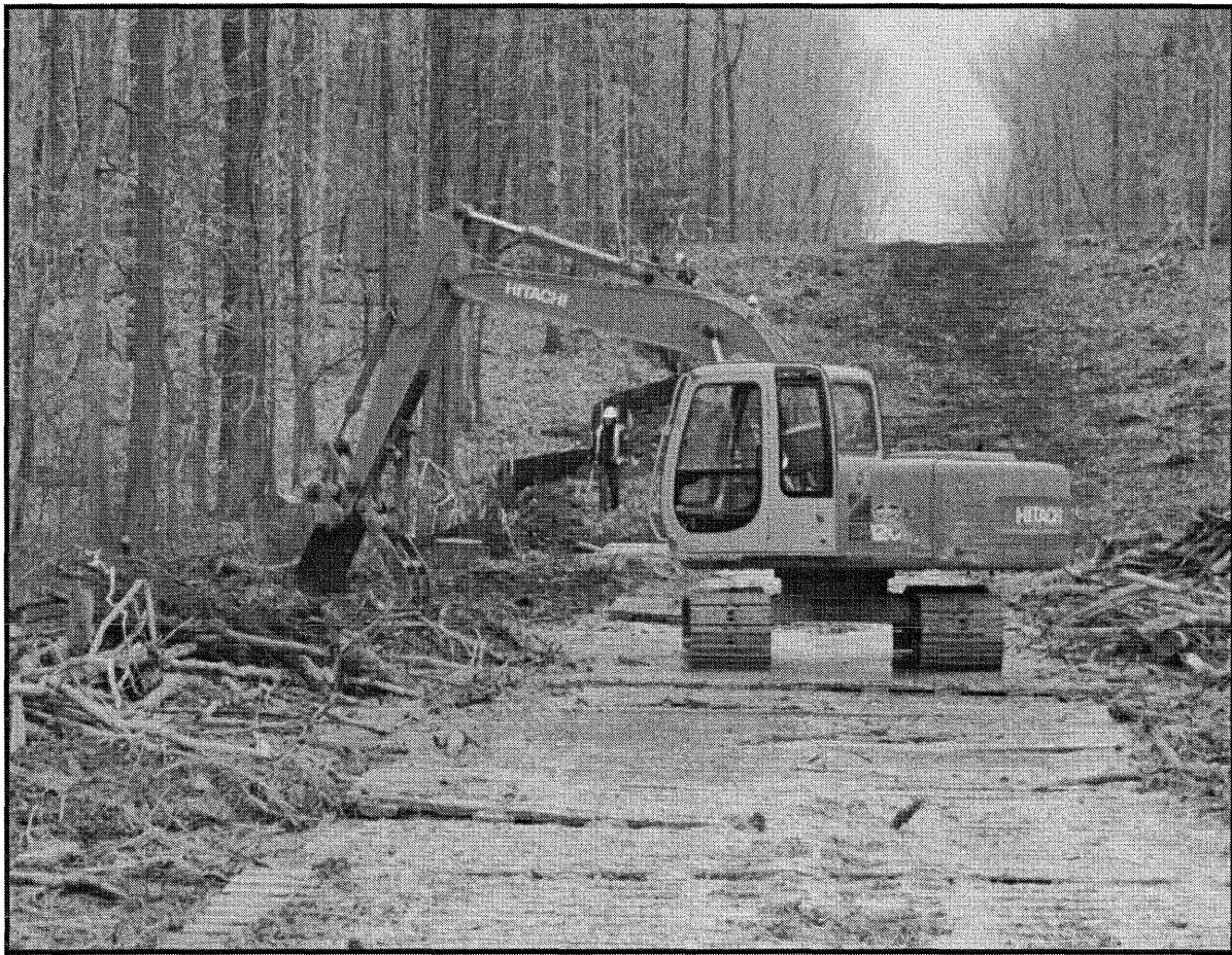
Figure 9: Right of way being cleared for Garrisonville underground project.
