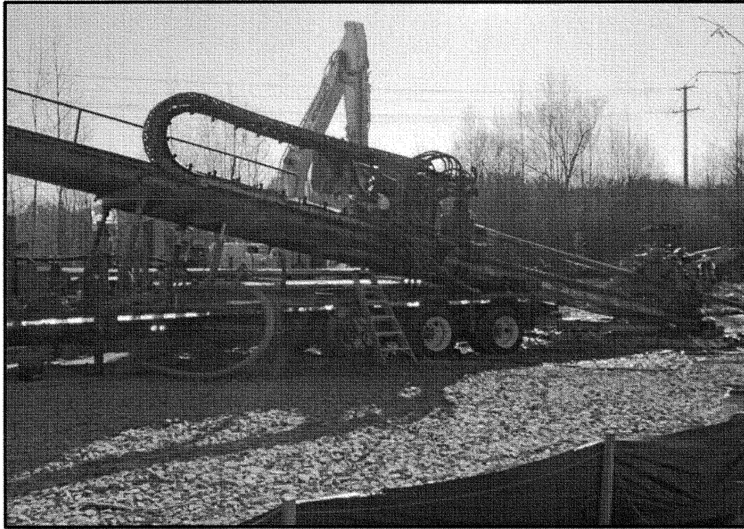
Figure 3: Horizontal Directional Drill Rig.
