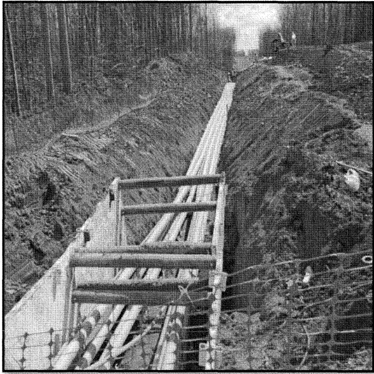
Figure 12: Construction of a portion of the Garrisonville line (trenched portion).
