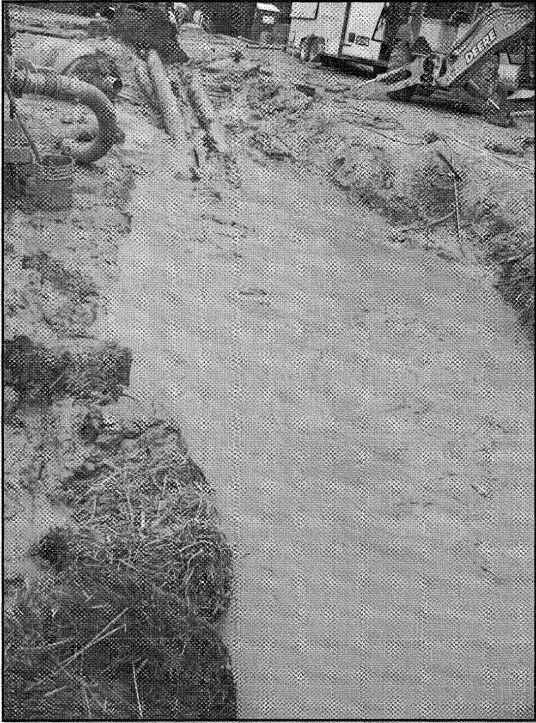
Figure 7: A picture of drilling mud at one termination of a drilling span.
