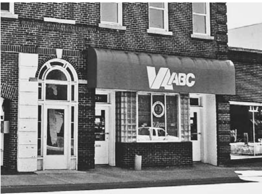
(Left) Opened on June 25, 1934, six months after the repeal of Prohibition, Virginia ABC Store 123 at 531 Main Street in Clifton Forge holds a unique place in ABC history as the only store to remain in its original location for 75 years. On the eve of the store's 75th anniversary, ABC Board Commissioners Susan Swecker and Frank Hall, and representatives from the Wholesale/Retail Division and Bureau of Law Enforcement hosted an open house focusing on Clifton Forge's unique place in ABC history and the agency's public safety mission.
