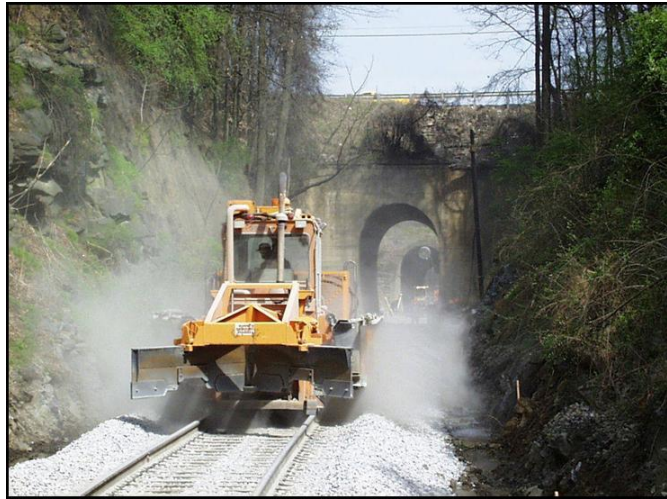
Photo Source: AREMA, IPRE Seminar, Module 7: Track and ROW Maintenance PowerPoint. Chicago. Sept. 2005
