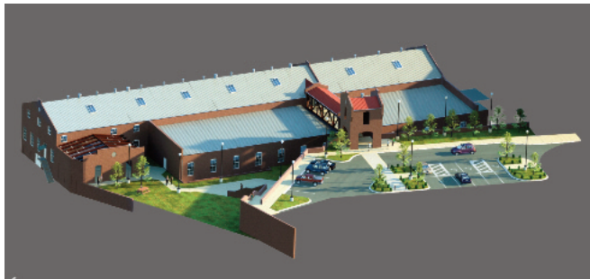
The R&D Center for Advanced Manufacturing and Energy Efficiency will be housed in a renovated historic tobacco facility located at the Southern Virginia Higher Education Center in Halifax County and will focus on advanced manufacturing techniques and a “Smart Factory” approach to demonstrate how emerging trends in industry can be adopted.
