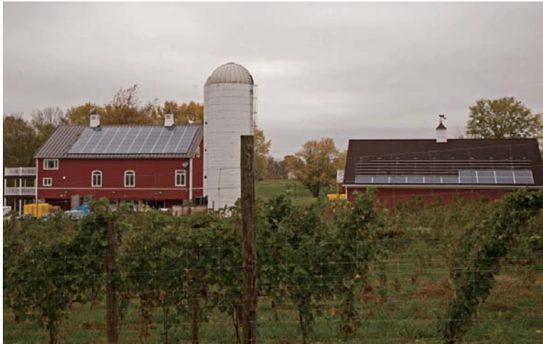
Virginia Green member Sunset Hills Vineyard completed the largest solar installation in Loudoun County in late 2010 (under construction above). It is sized to replace 100% of the winery's electrical usage.
