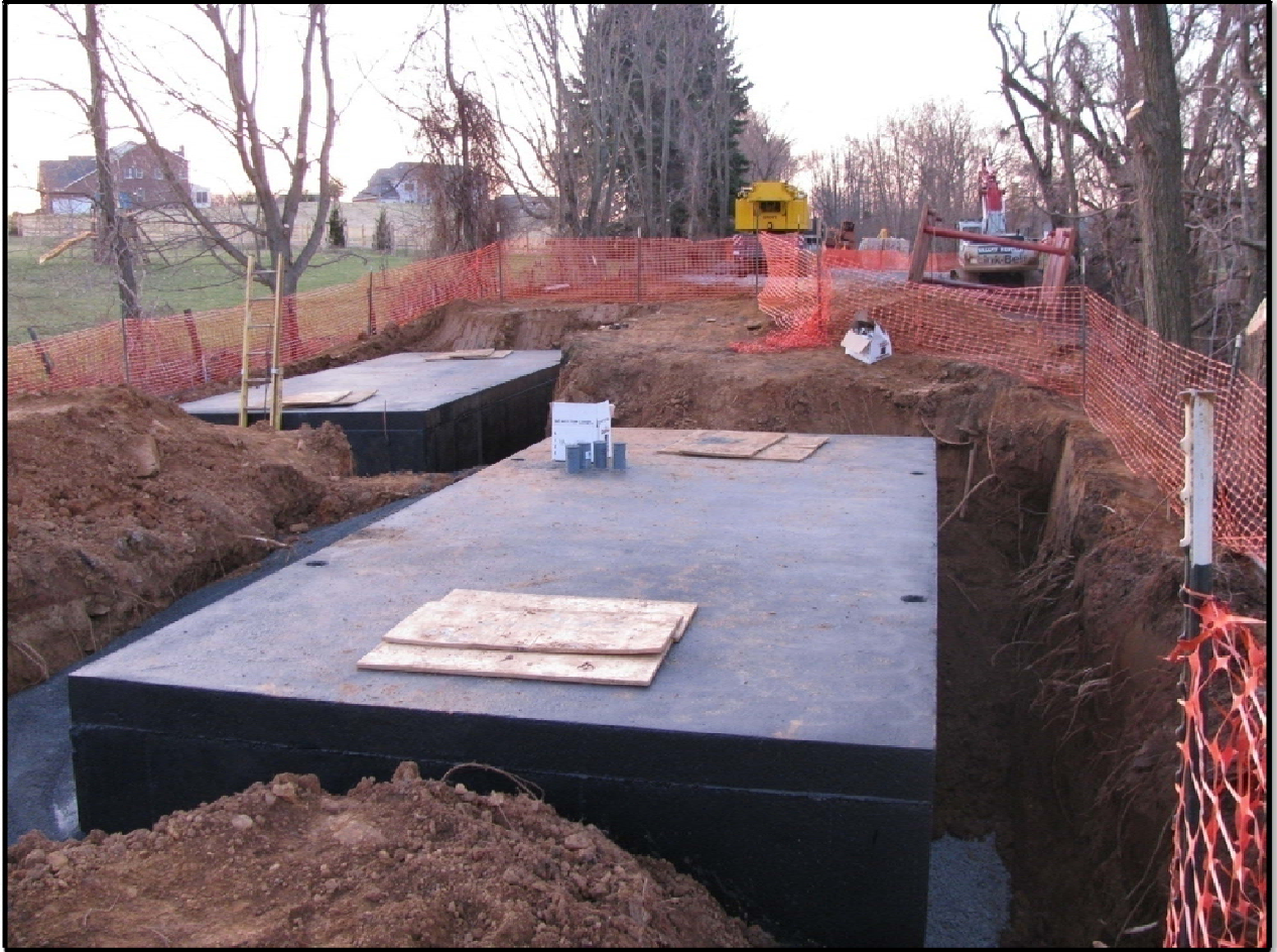
Figure 2: Manholes "6A" and "6B." Once restored, the W&OD Trail will thread between the four manhole lids on the surface.
