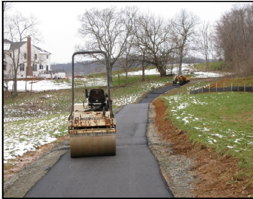
Figure 1: Paving the Detour Trail; before construction began in January 2010.
