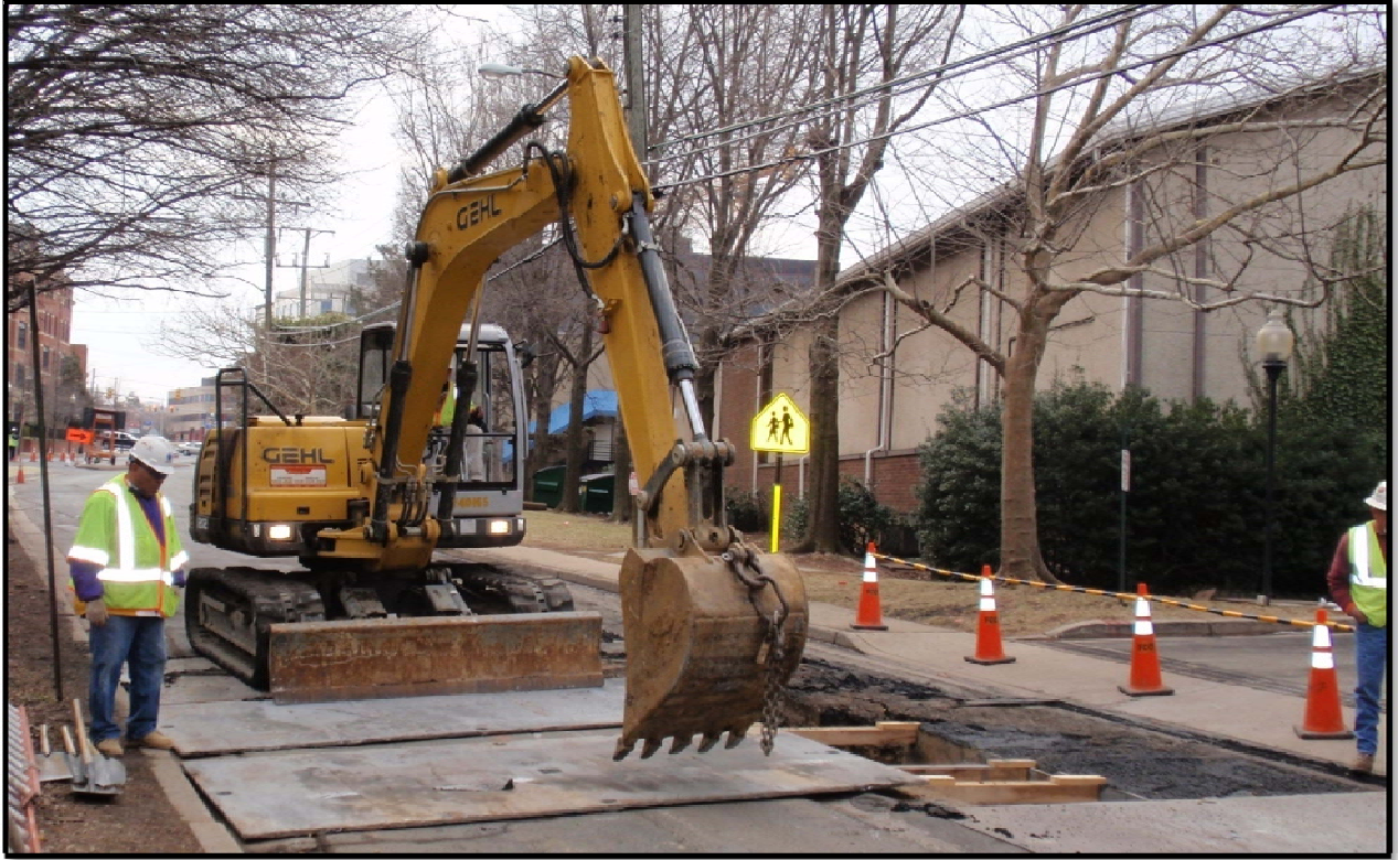
Figure 12: Excavation for Clarendon -- Ballston underground transmission line.
