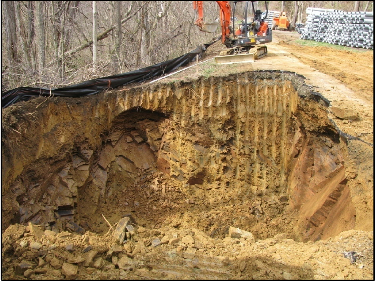
Figure 4: Layers of dense rock below and beside the original trail (top right). Stacks of conduit (pipe) also visible.
