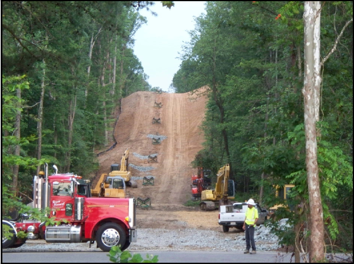
Figure 14: Cleared right of way for Garrisonville project.
