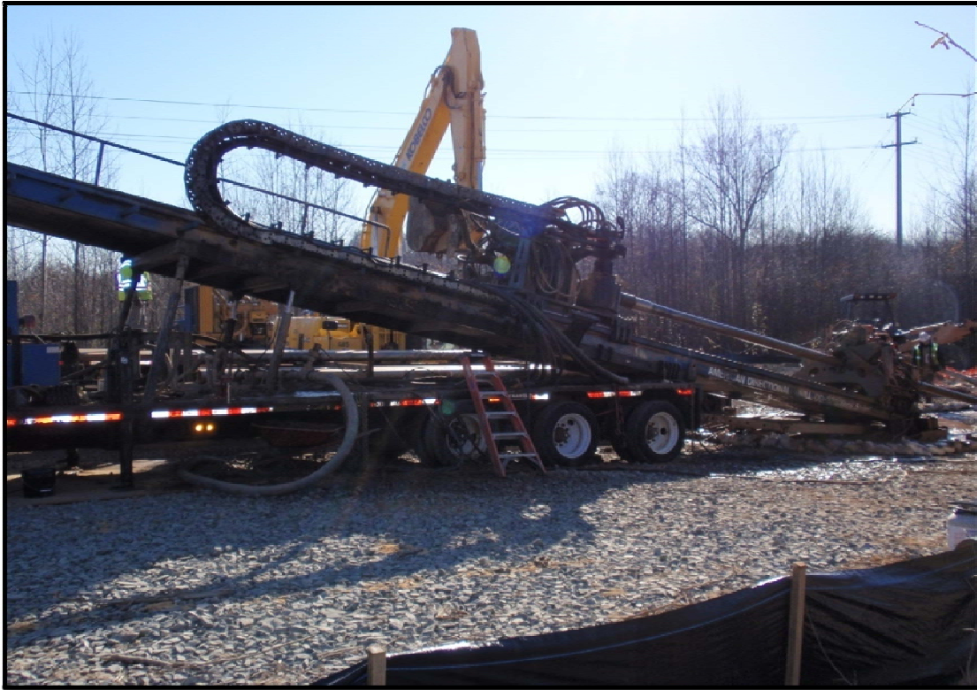
Figure 7: Horizontal Directional Drill Rig.
