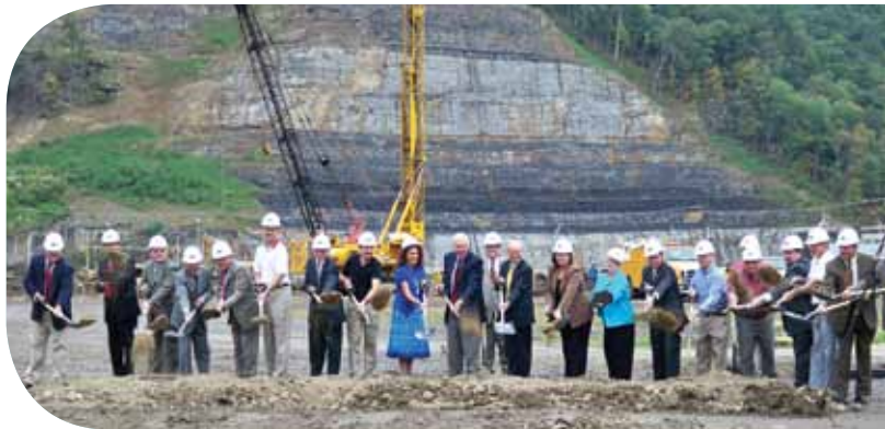
VCEDA joins Congressman Rick Boucher, the Town of Grundy and regional officials for the groundbreaking of the town's new retail center to be the anchor of a 13-acre redevelopment site. VCEDA approved a $2 million grant to the IDA of the Town of Grundy to be used for the construction of a 500-car parking facility, which will be the base for a major retail center to be built on top of the garage. VCEDA also approved up to a $1 million grant and a $1.5 million loan to assist with the Grundy redevelopment project in 2000.
