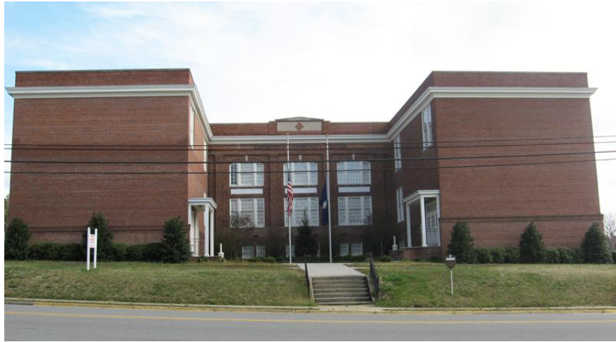
Figure 11: Kenbridge Community Center, Lunenburg County
