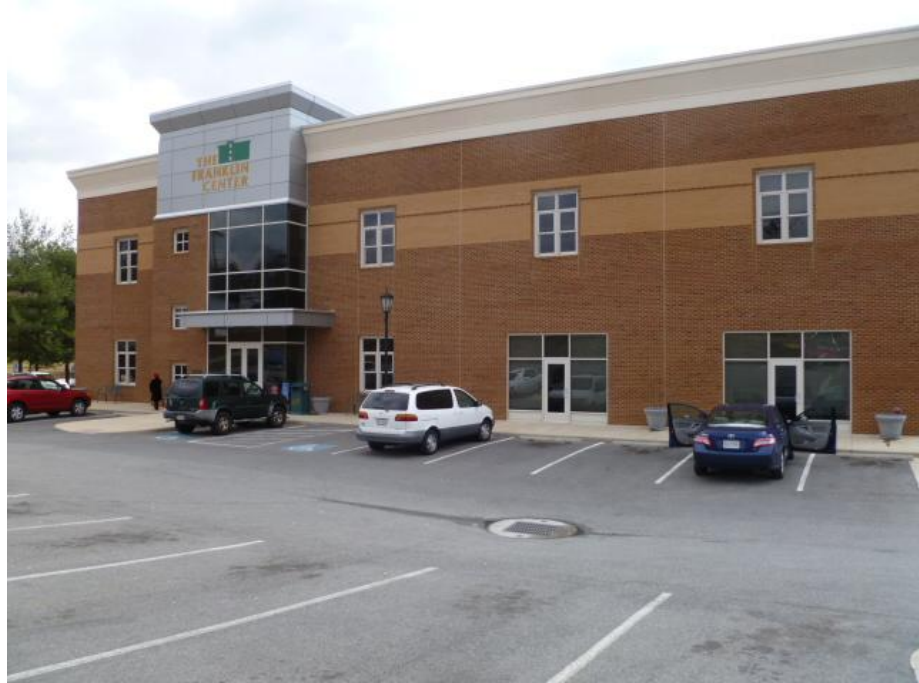
Figure 8: Franklin Center for Advanced Learning and Enterprise, Franklin County
