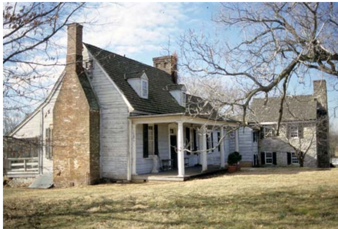
Clermont Farm, Clarke Co.: In 2004, the 361-acre Clermont property, which is managed as a working farm and living museum by The Clermont Trust, was bequeathed to DHR by Elizabeth Rust Williams' estate.
