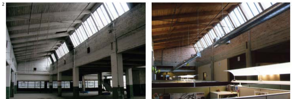
[2-3] Clerestory windows provide natural light in a historic industrial building: Before and after rehabilitation.
