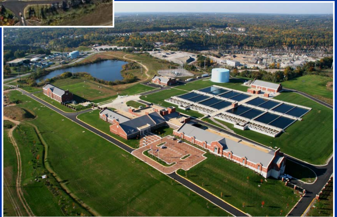
7. Low Southwest view of Griffith WTP 10-21-06
