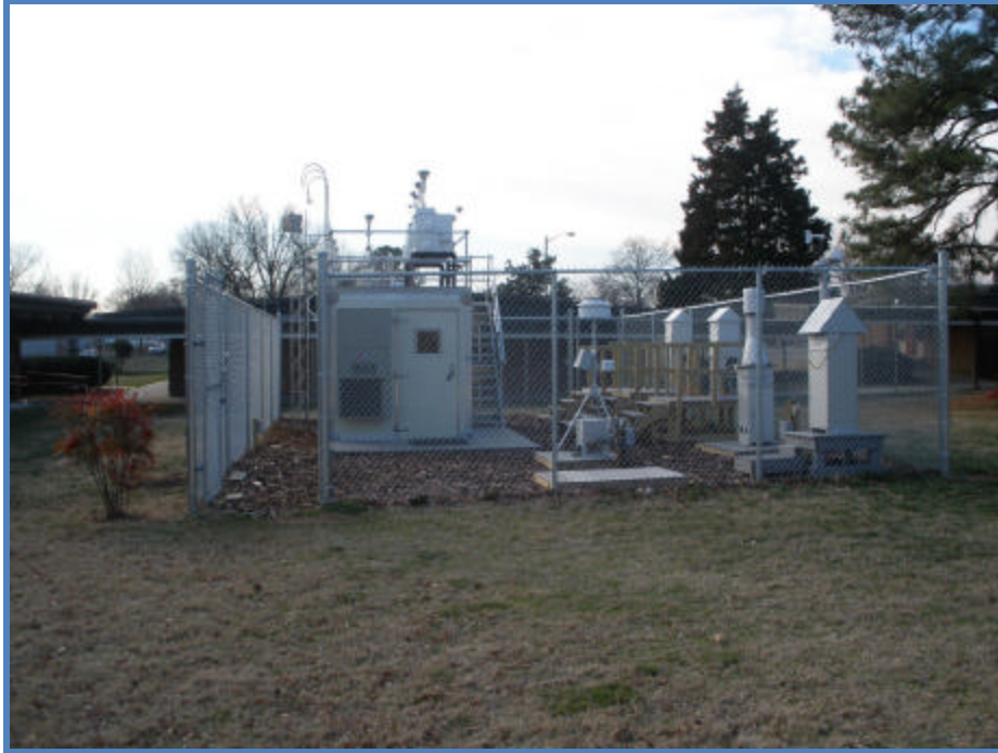
Figure 2-2: View of the Henrico County NATTS/NCORE Site Looking South
