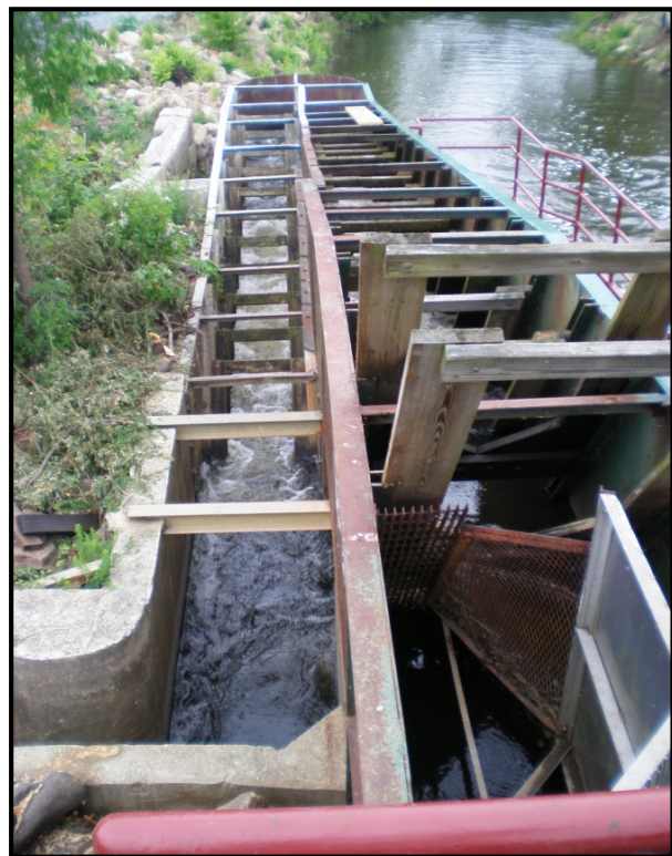
Figure 7 Photo of Baffled Chutes
