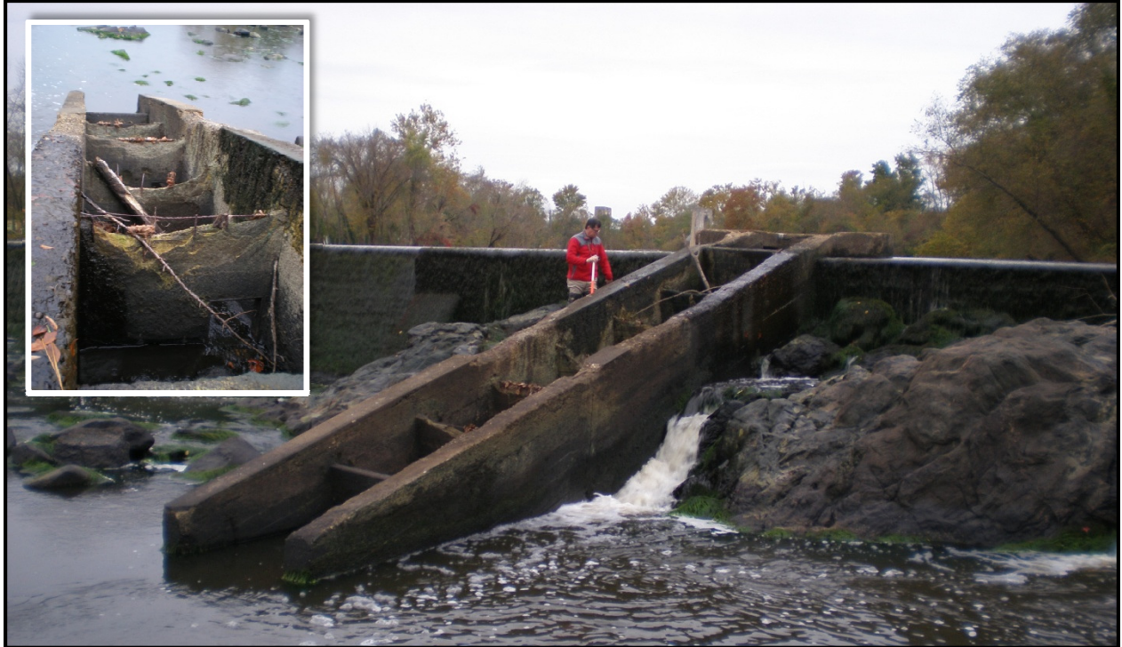
Figure 13 Pool and Weir Fishway near Center of Dam
