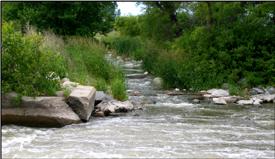
Figure 16 Nature-Like Bypass Channel (Photo courtesy of Dr. Luther Aadland)
