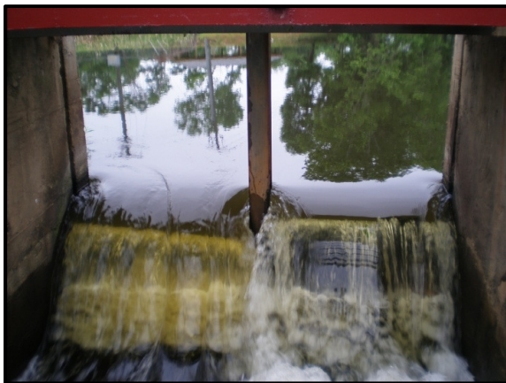
Figure 4 Photo of Attraction Flow Inlet from Reservoir
