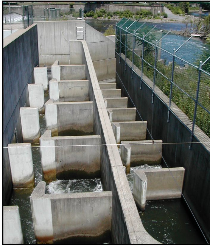
Figure 15 Vertical Slot Fishway at Easton Dam on the Lehigh River, PA
