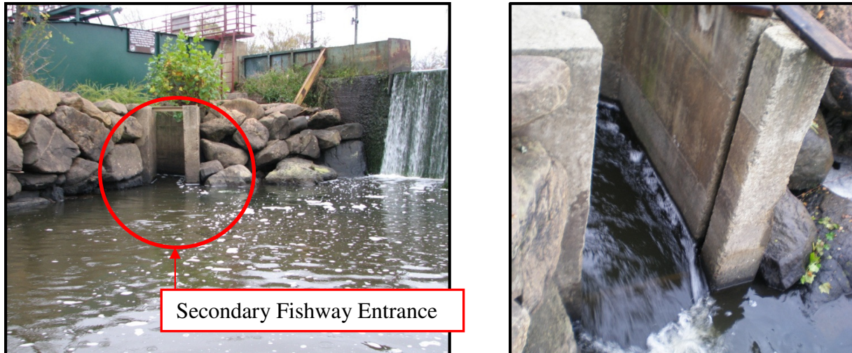
Figure 3 Secondary (Upper) Fishway Entrance at Right Abutment of Spillway
