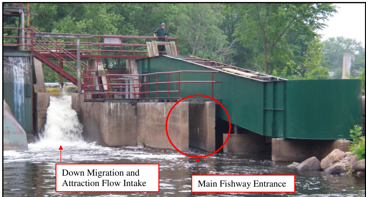
Figure 2 Main (Lower) Fishway Entrance in Siphon Tailrace
