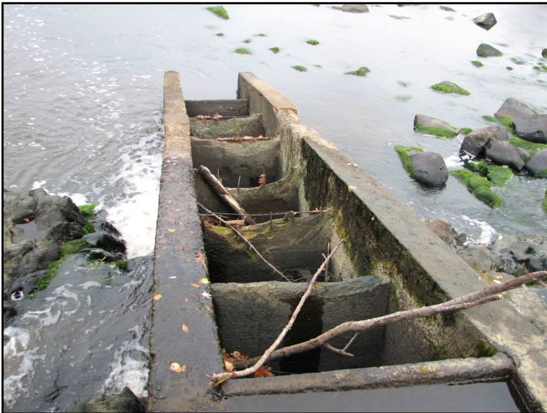
Pool and Weir Fishway near Center of Harvell Dam
