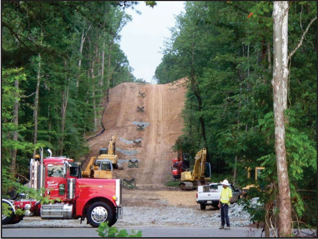
Figure 14: Cleared right of way for Garrisonville project.
