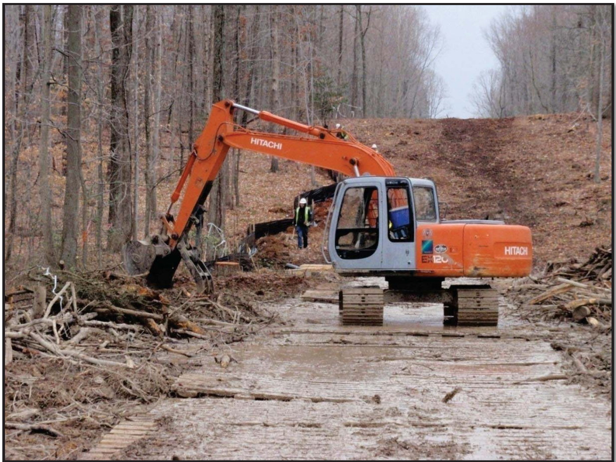
Figure 13: Right of way being cleared for Garrisonville underground project.
