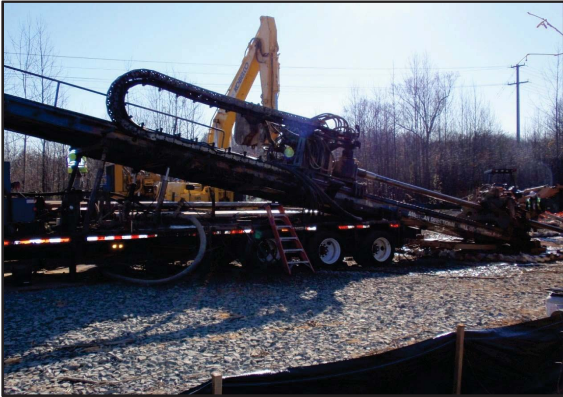
Figure 7: Horizontal Directional Drill Rig.
