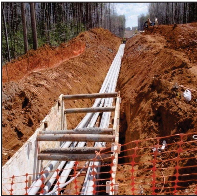
Figure 16: Construction of a portion of the Garrisonville line (trenched portion).
