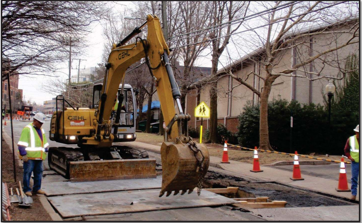
Figure 12: Excavation for Clarendon -- Ballston underground transmission line.
