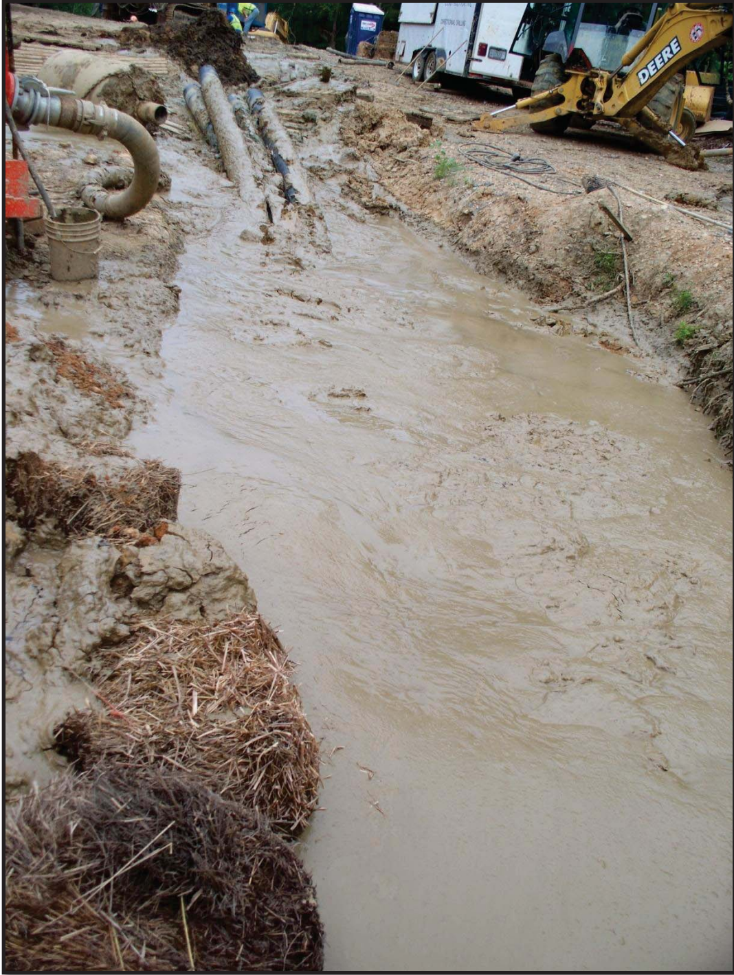
Figure 11: A picture of drilling mud at one termination of a drilling span.
