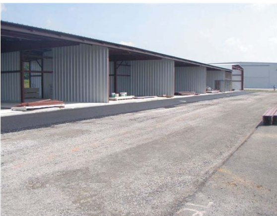
T-hanger construction in progress
