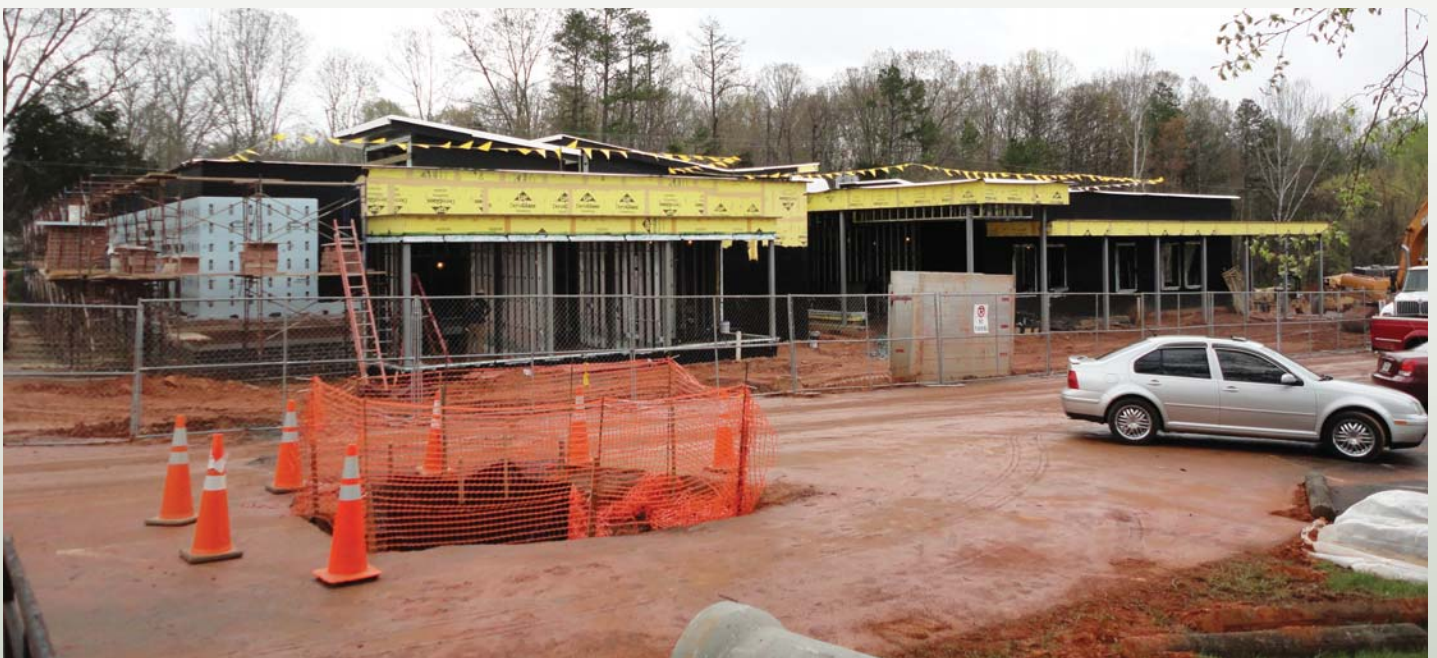
Administrative Building Under Construction
