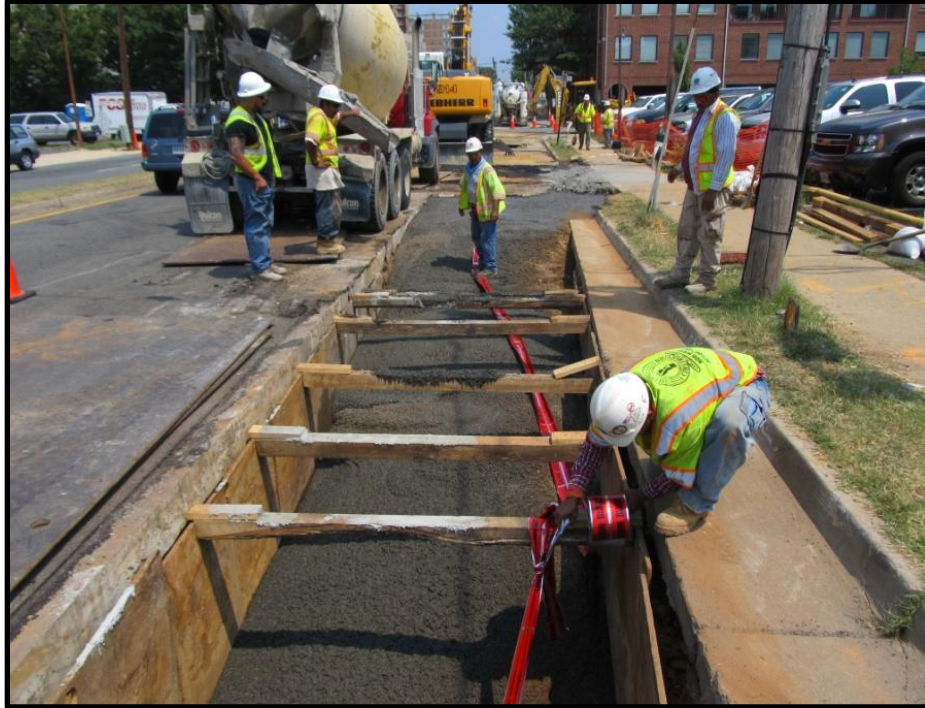
Figure 1: Crews utilize right lane of traffic to underground line.
