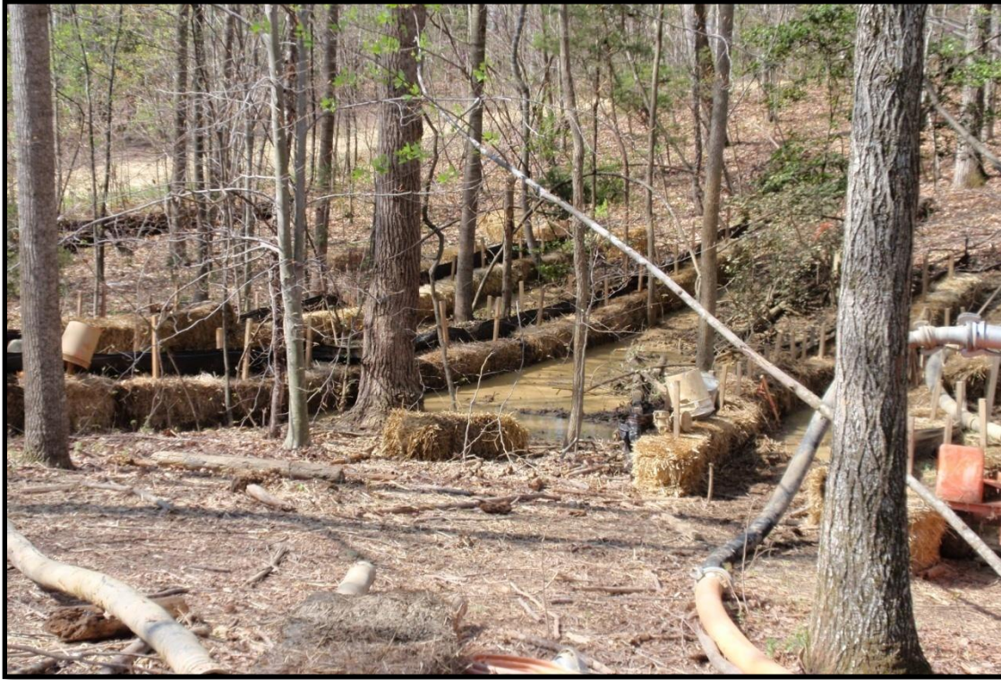
Figure 11: Site of frac-out showing containment measures for the protection of the environment.
