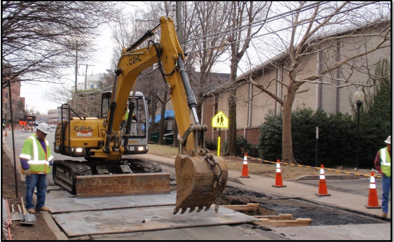
Figure 14: Excavation for Clarendon -- Ballston underground transmission line.
