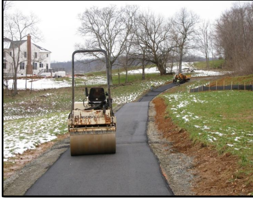
Figure 3: Paving the Detour Trail; before construction began in January 2010.
