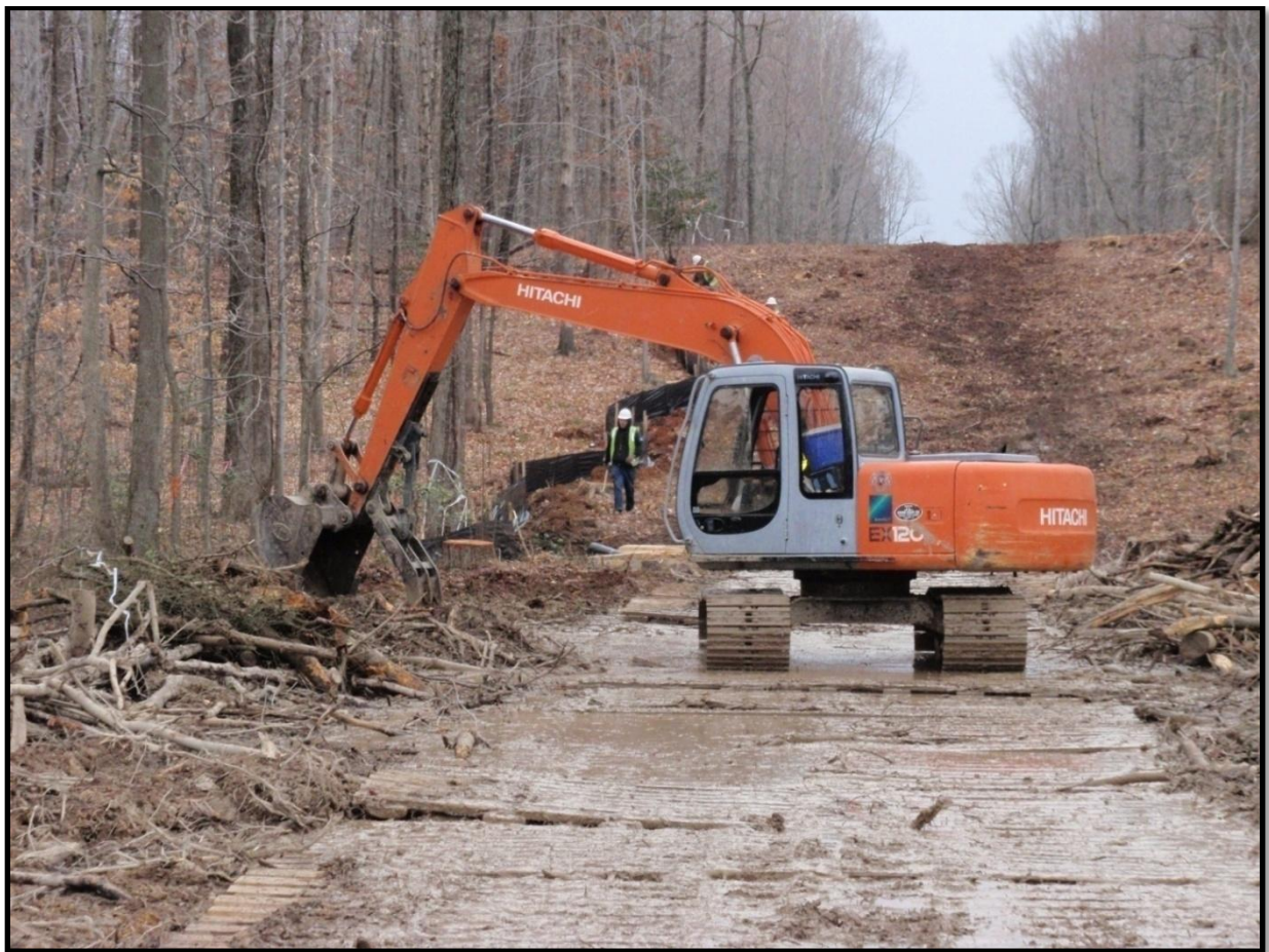
Figure 15: Right of way being cleared for Garrisonville underground project.
