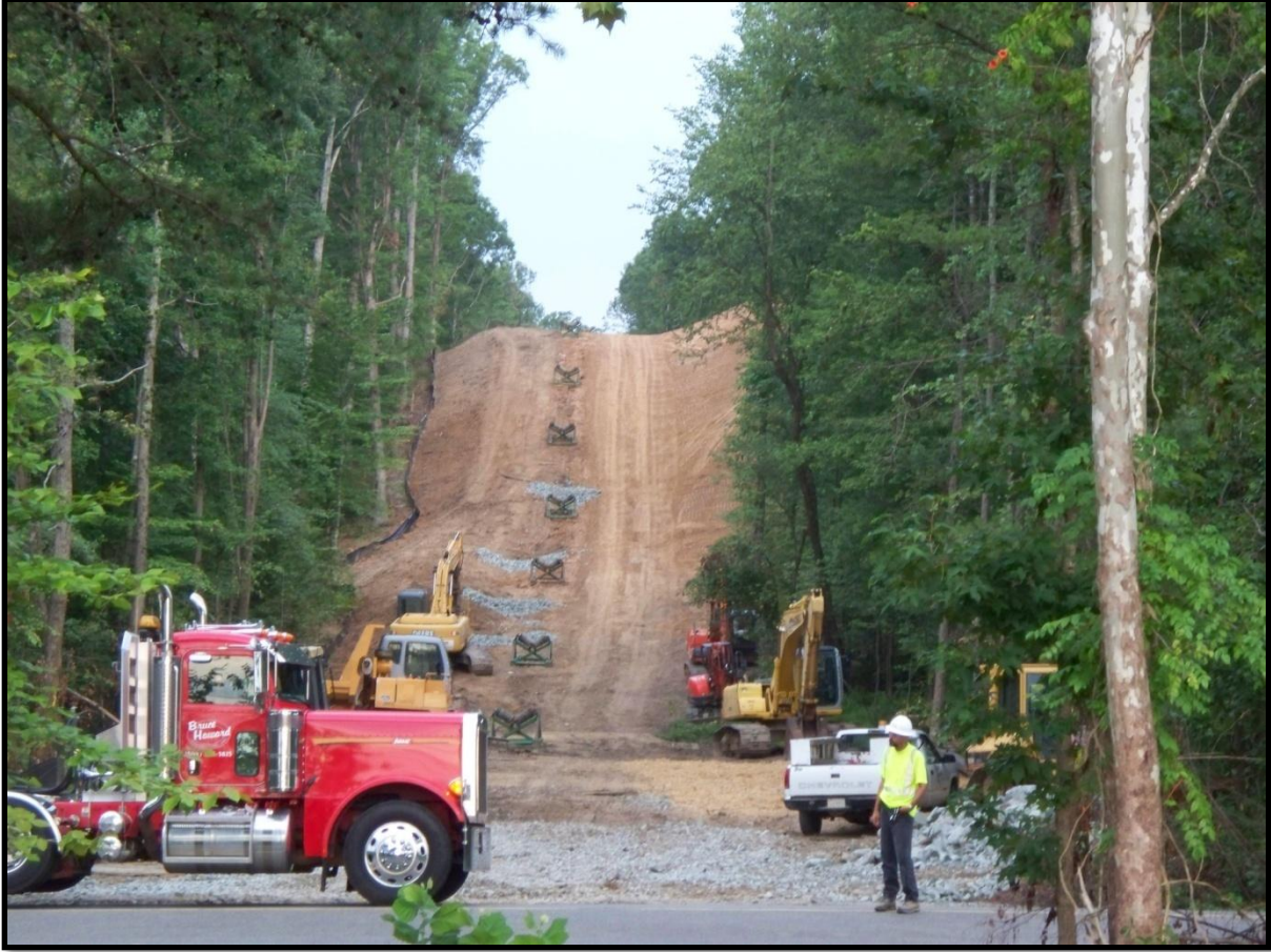
Figure 16: Cleared right of way for Garrisonville project.
