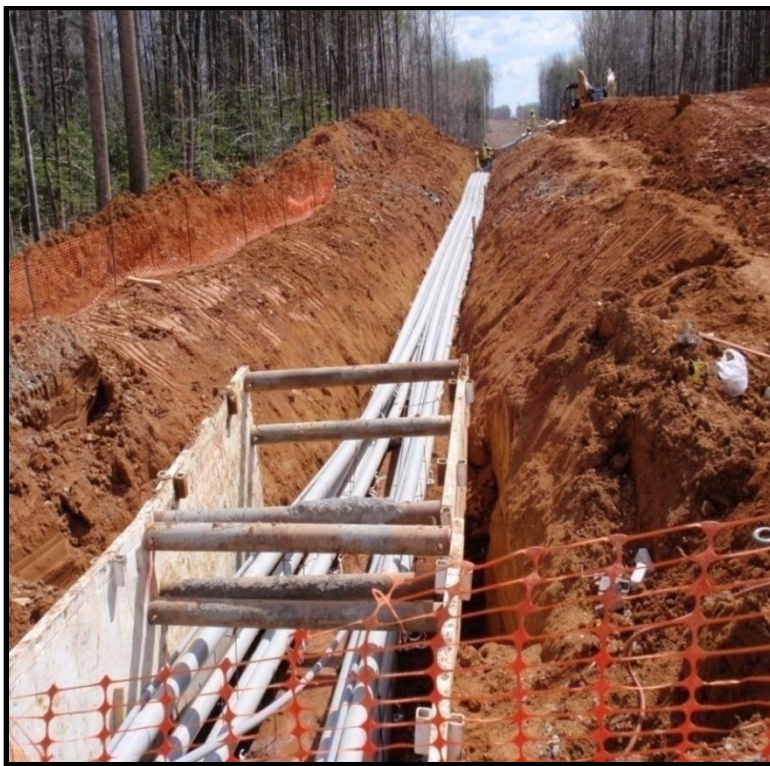
Figure 18: Construction of a portion of the Garrisonville line (trenched portion).
