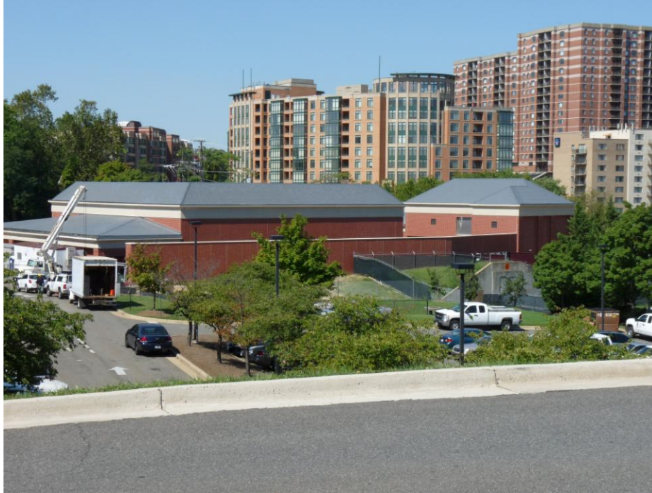
Figure 2: Completed Radnor Heights Substation is consistent with community aesthetics.
