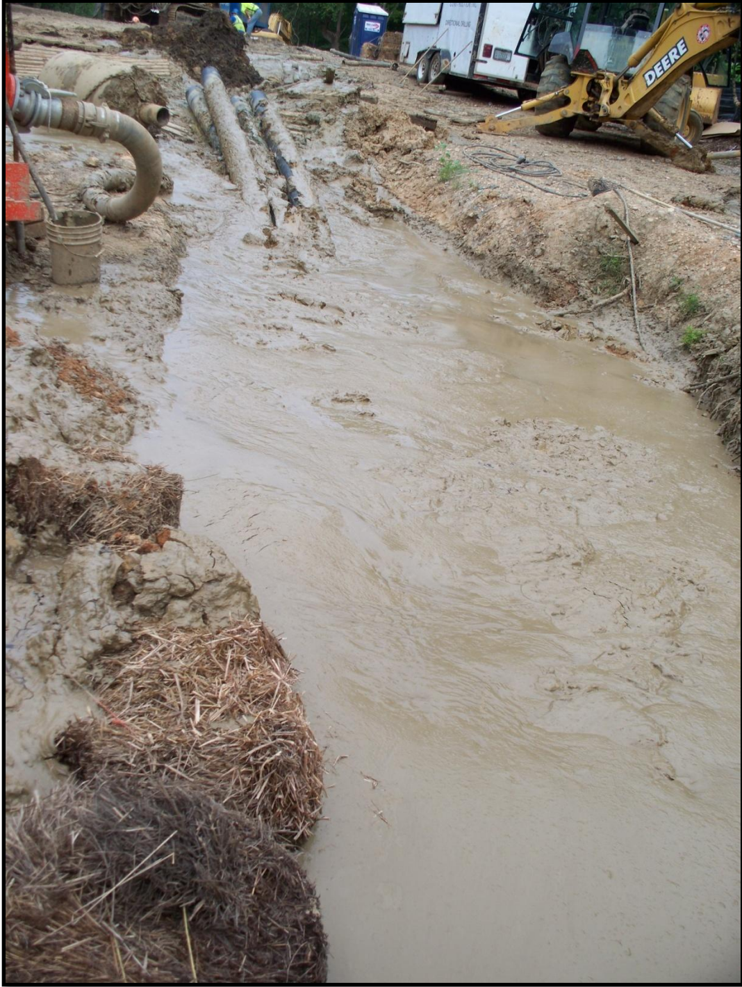
Figure 13: A picture of drilling mud at one termination of a drilling span.
