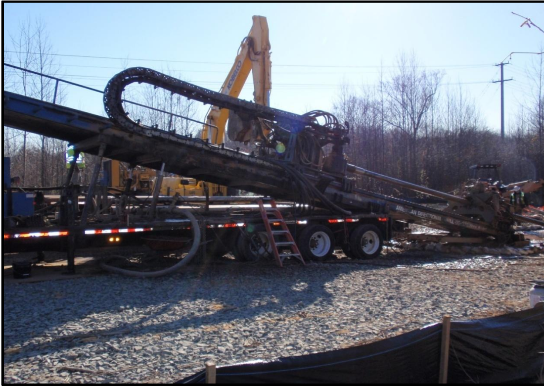
Figure 9: Horizontal Directional Drill Rig.
