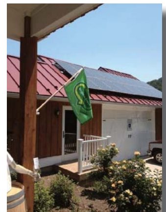
Solar panels at DuCard Vineyards, a Virginia Green member
