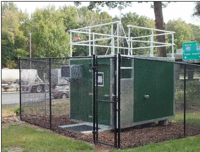
Figure 2-2: Bryan Park Near-Road Monitoring Site
