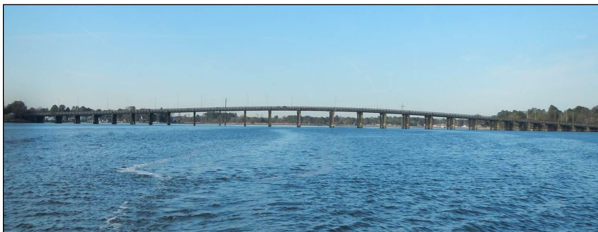
Figure 3 - Churchland Bridge as viewed from the Western Branch of the Elizabeth River.
