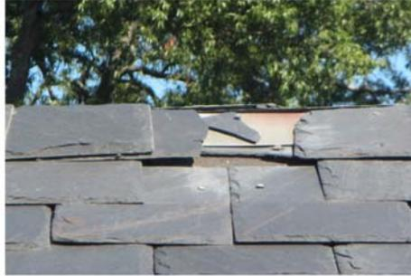
Brick buildings may develop cracked or failing mortar joints, which may lead to water infiltration or structural damage. Aging roofs can leak, potentially damaging a facility's interior, including research or instructional equipment. Brickwork (left) is cracked, and slate roof (right) is 30 years past its expected useful life of 50 years (Rollins Hall, ODU).
