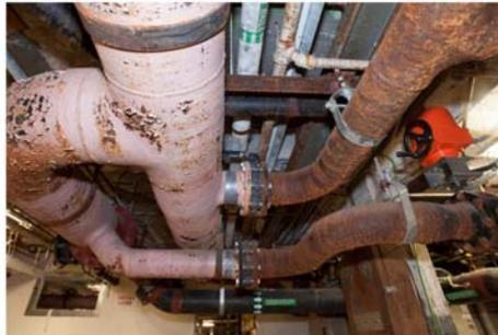
Systems past their useful expected life may be at risk of failure. Air handler (left) uses refrigerants no longer approved by the EPA (Koch Hall, ODU). Building (right) contains deteriorated chilled water piping (West Hospital, VCU).
