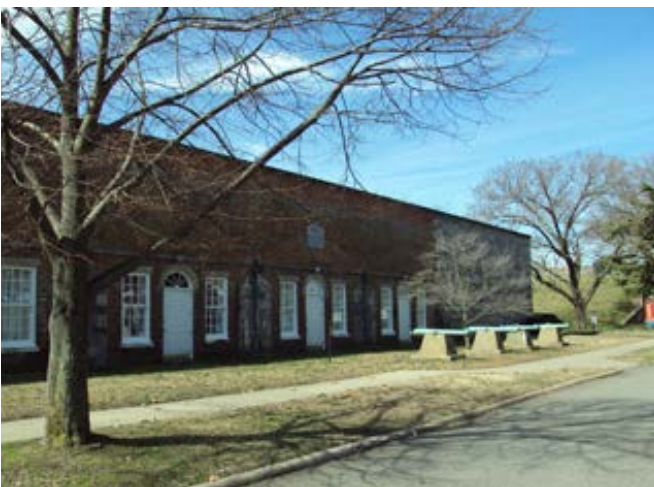
Part of the casemate that forms the Stone Fort at Fort Monroe. (Photos: DHR)
