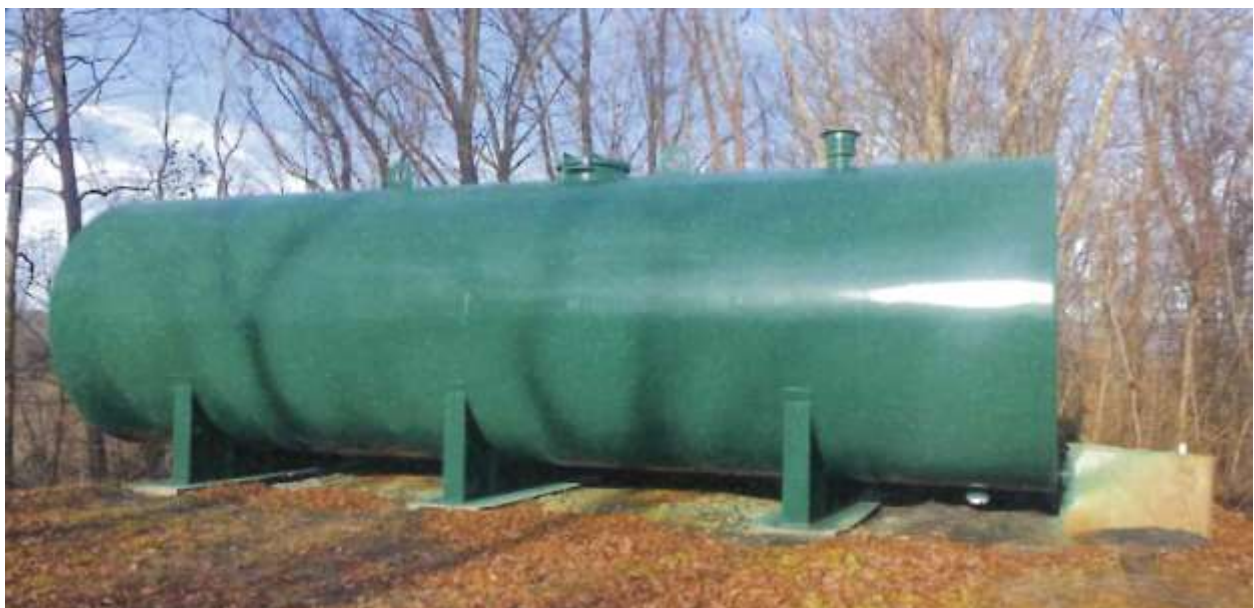
St. Paul - Hardy Hollow Tank – After
