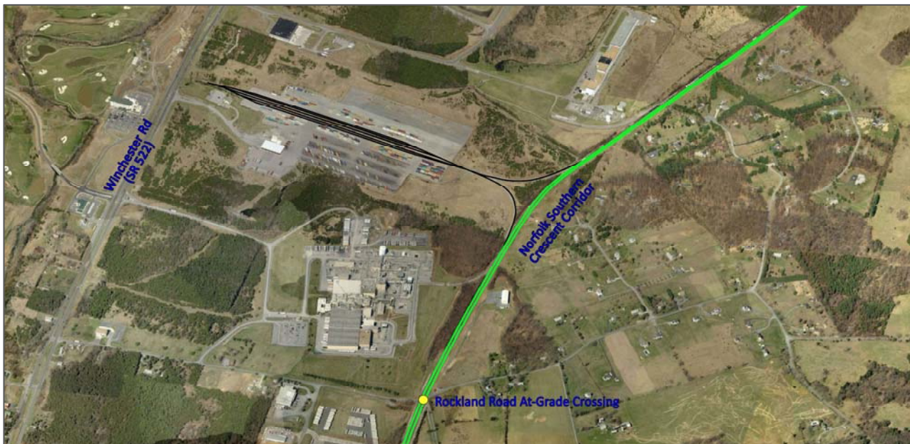
Figure 26 – VIP On-Dock Rail System
