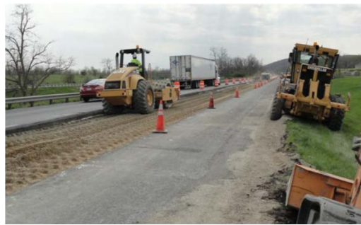
Full Depth Reclamation
