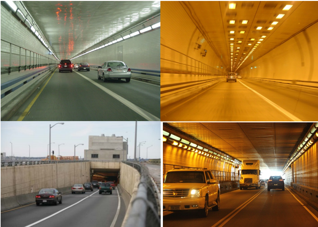
Figure 17: Virginia Tunnel Facilities
