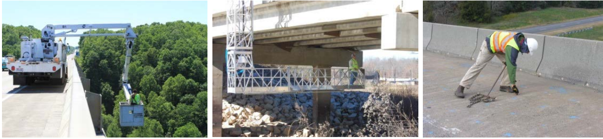
Figure 10: Bridge Condition Assessment
