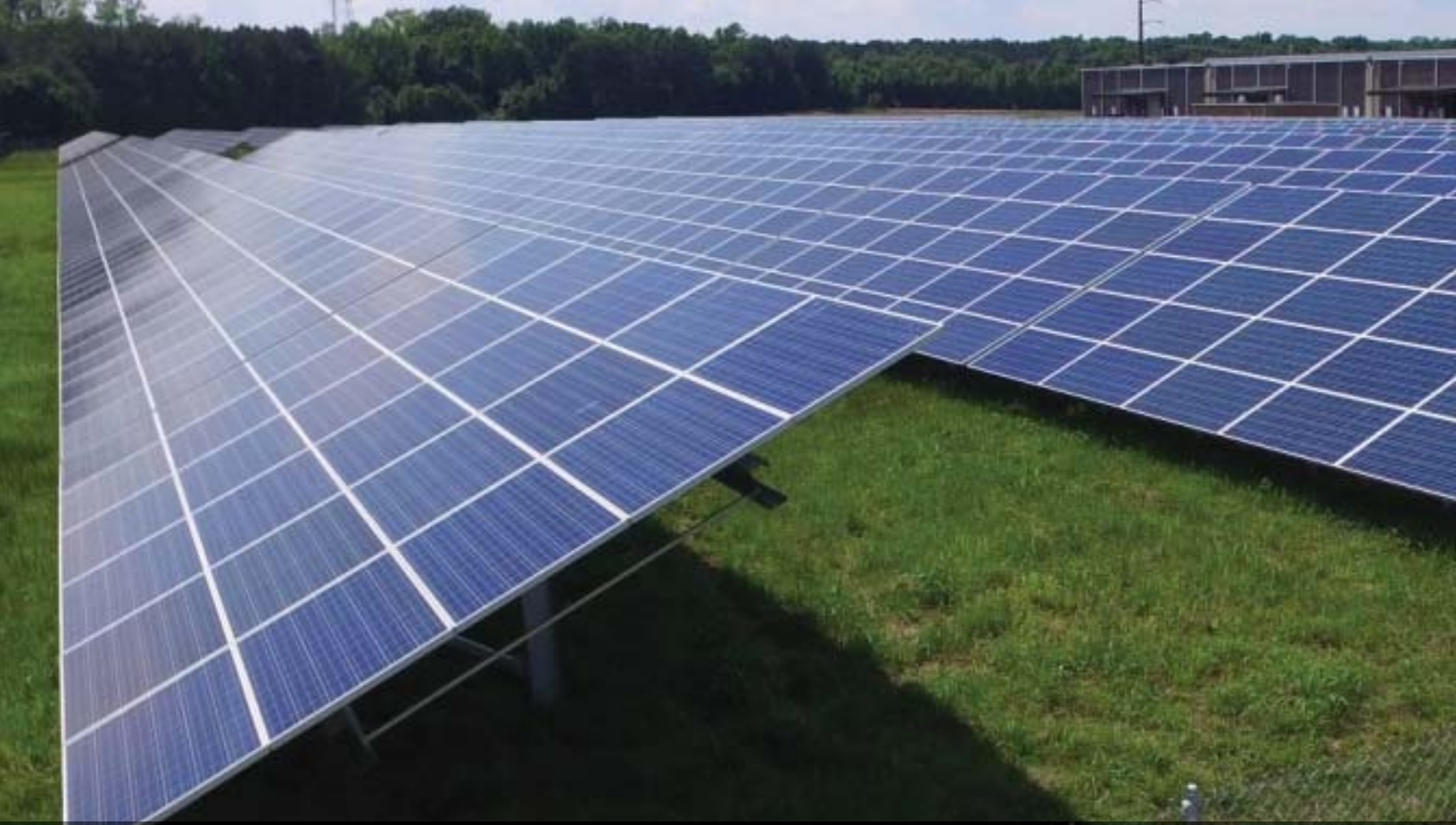
2000 KW AC ground mounted solar array installed at Philip Morris' Park 500 facility on Bermuda Hundred Road PHOTO CREDIT: DOMINION VIRGINIA POWER
