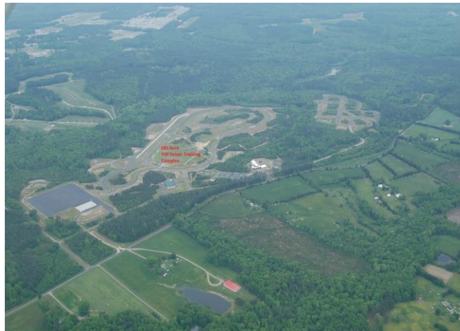
Figure 1: Aerial View of DTC
