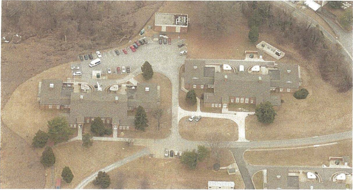
AERIAL VIEW SOUTH OF BUILDINGS 11 AND 12
