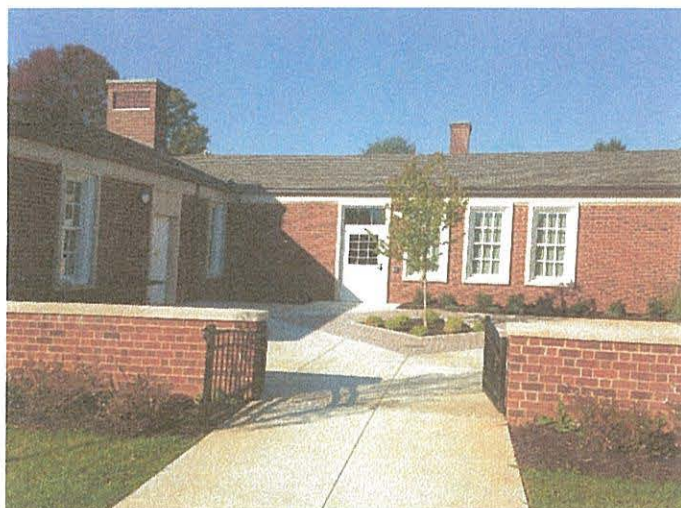
Typical Asphalt Roof Shingles with Aluminum Gutters and Downspouts
