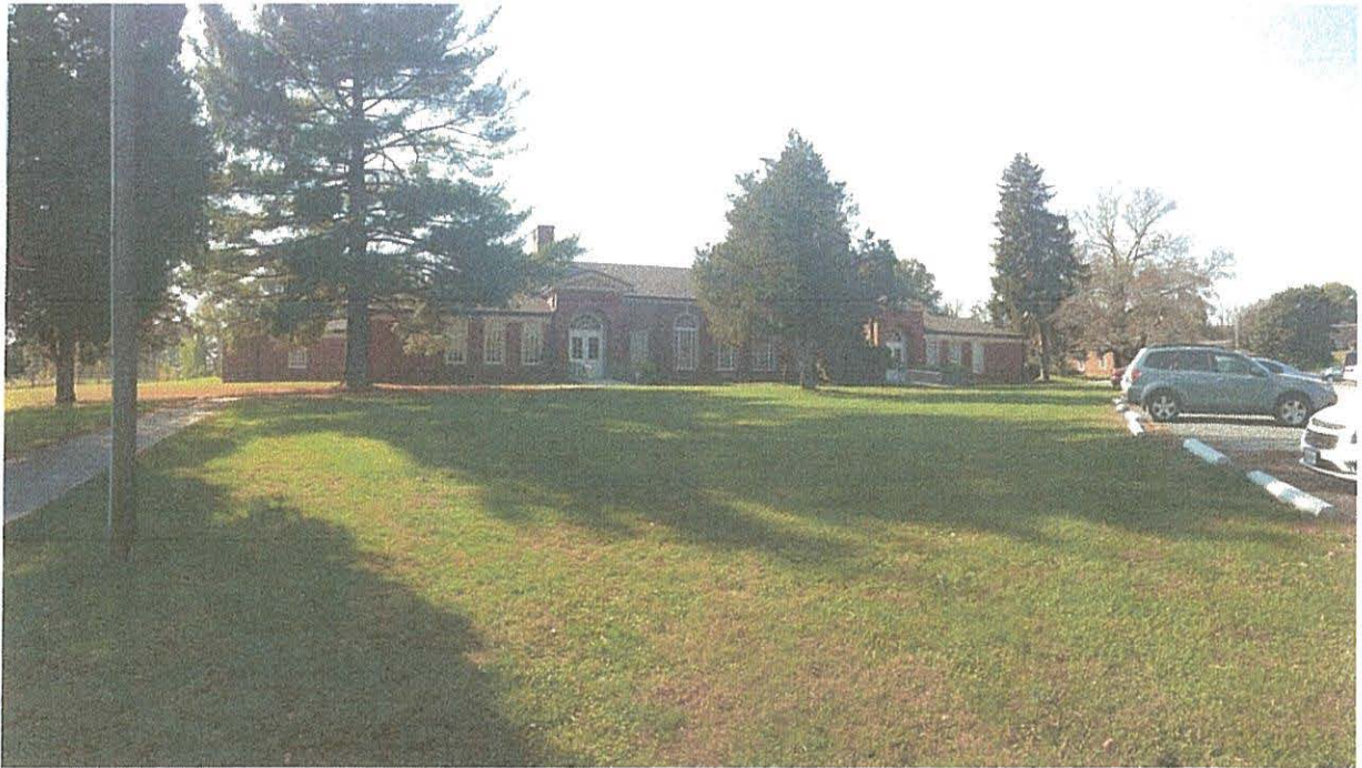
FRONT VIEW OF BUILDING 11
