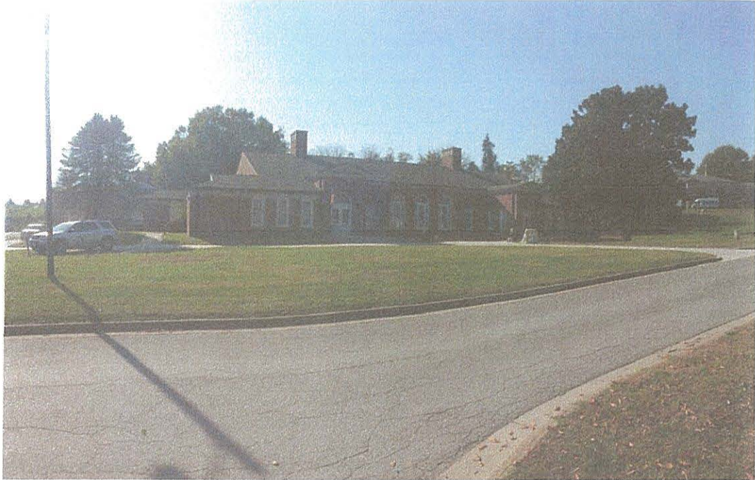
FRONT VIEW OF BUILDING 12
