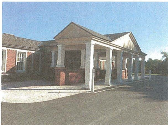
Wood Trim at Building 10 – Columns, Eaves, Soffits, Fascia, and Window Trim
