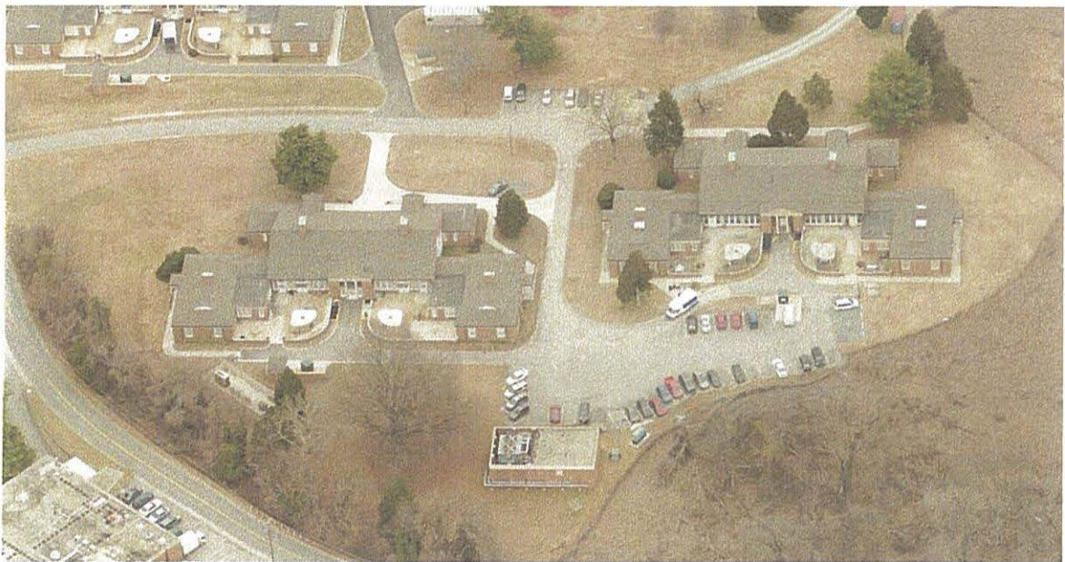
AERIAL VIEW NORTH OF BUILDINGS 11 AND 12
