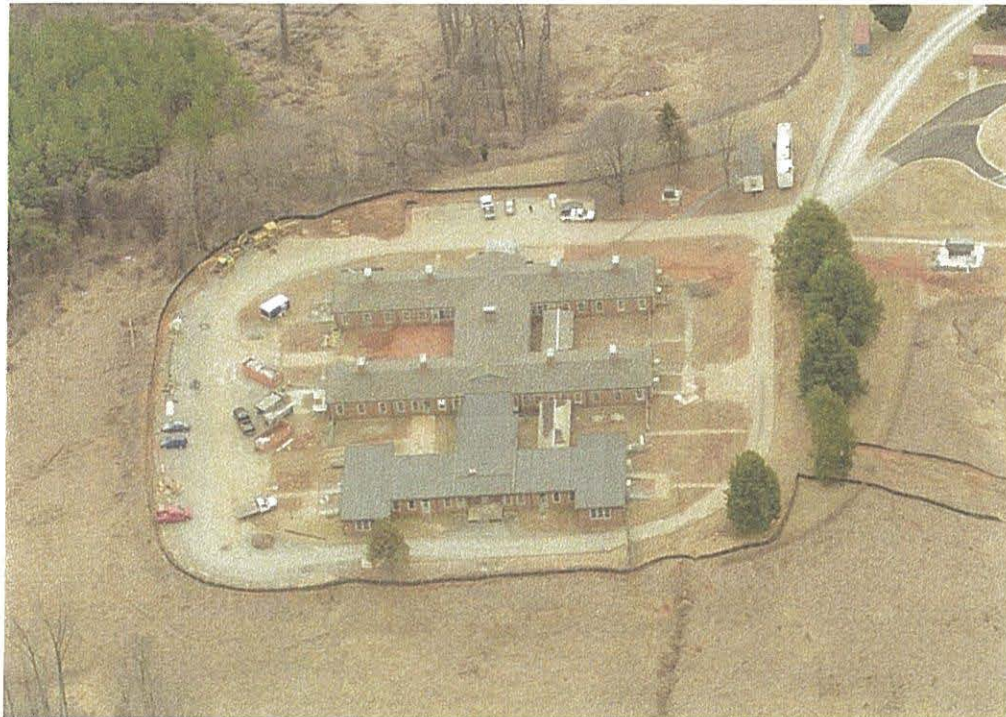
AERIAL VIEW SOUTH OF BUILDING 10 GREYLOCK ADVISORY GROUP, LTD.
