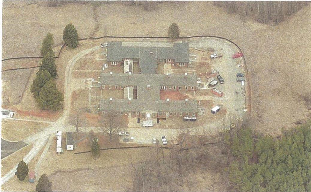
AERIAL VIEW NORTH OF BUILDING 10 (DURING RENOVATION)
