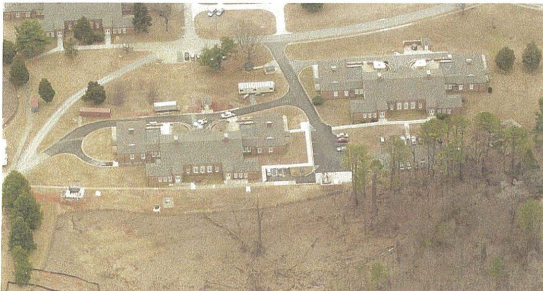
AERIAL VIEW SOUTH OF BUILDINGS 8 AND 9
