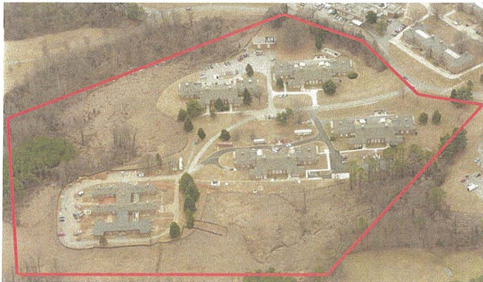
AERIAL VIEW SOUTH OF SUBJECT PROPERTY (LINES ABOVE ARE APPROXIMATE)
