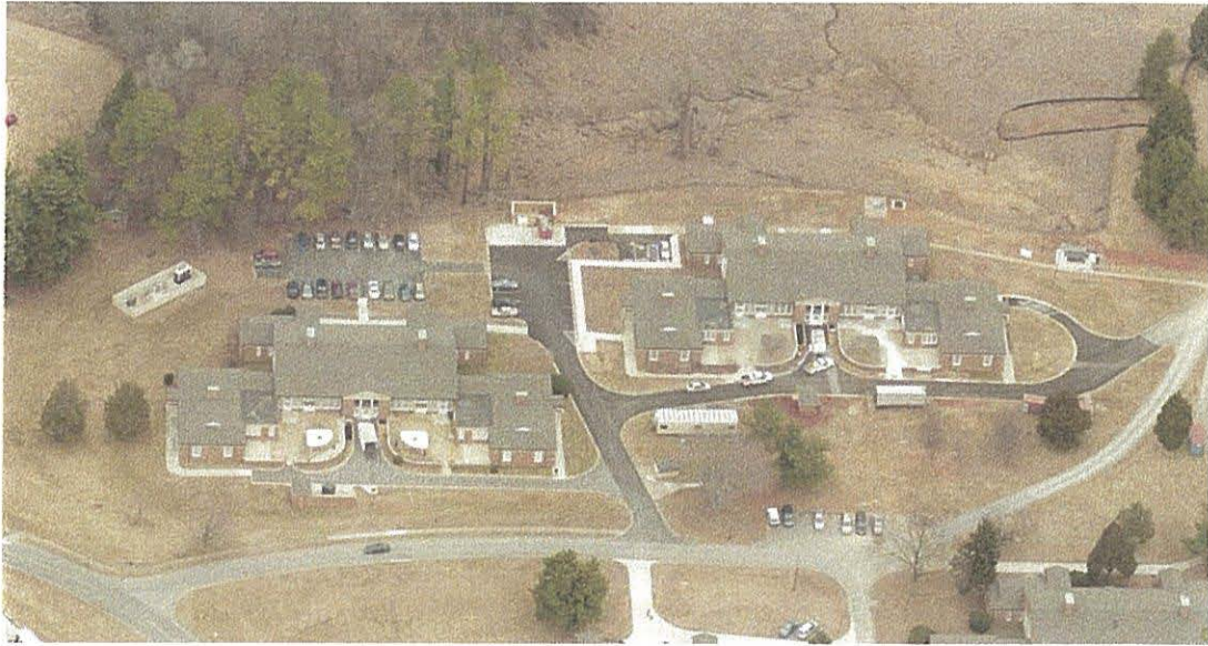
AERIAL VIEW NORTH OF BUILDINGS 8 AND 9
